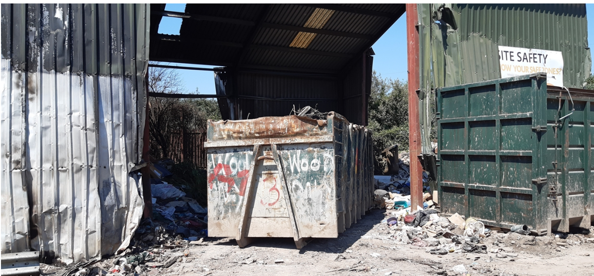
Photo 5 - Photo of fire incident taken by NRW Officer Greg GARDNER on 13/06/23
