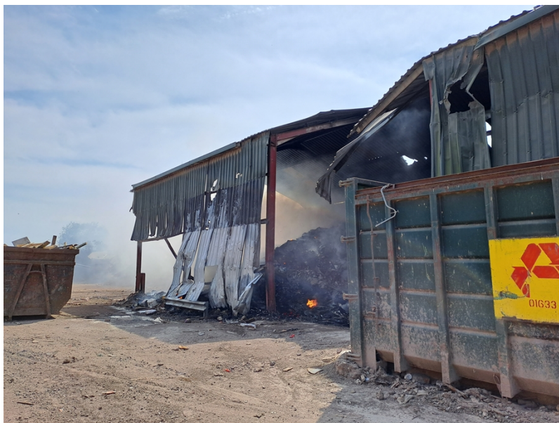
Photo 1 - Photo of fire incident taken by NRW Officer Alastair KRZYZOSIAK on 09/06/23
