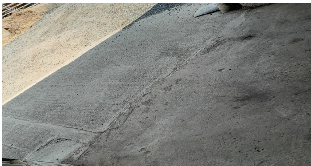
Photo 2 – doorway requiring raised lip for secondary containment
