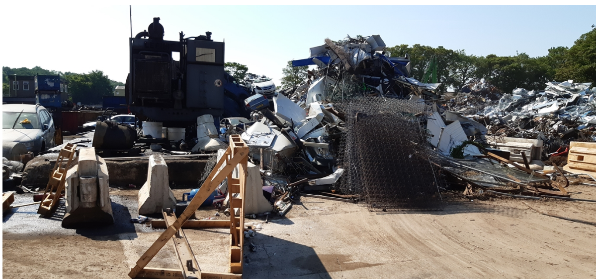
Photo 2 - Area where flooring infrastructure improvements have taken place
