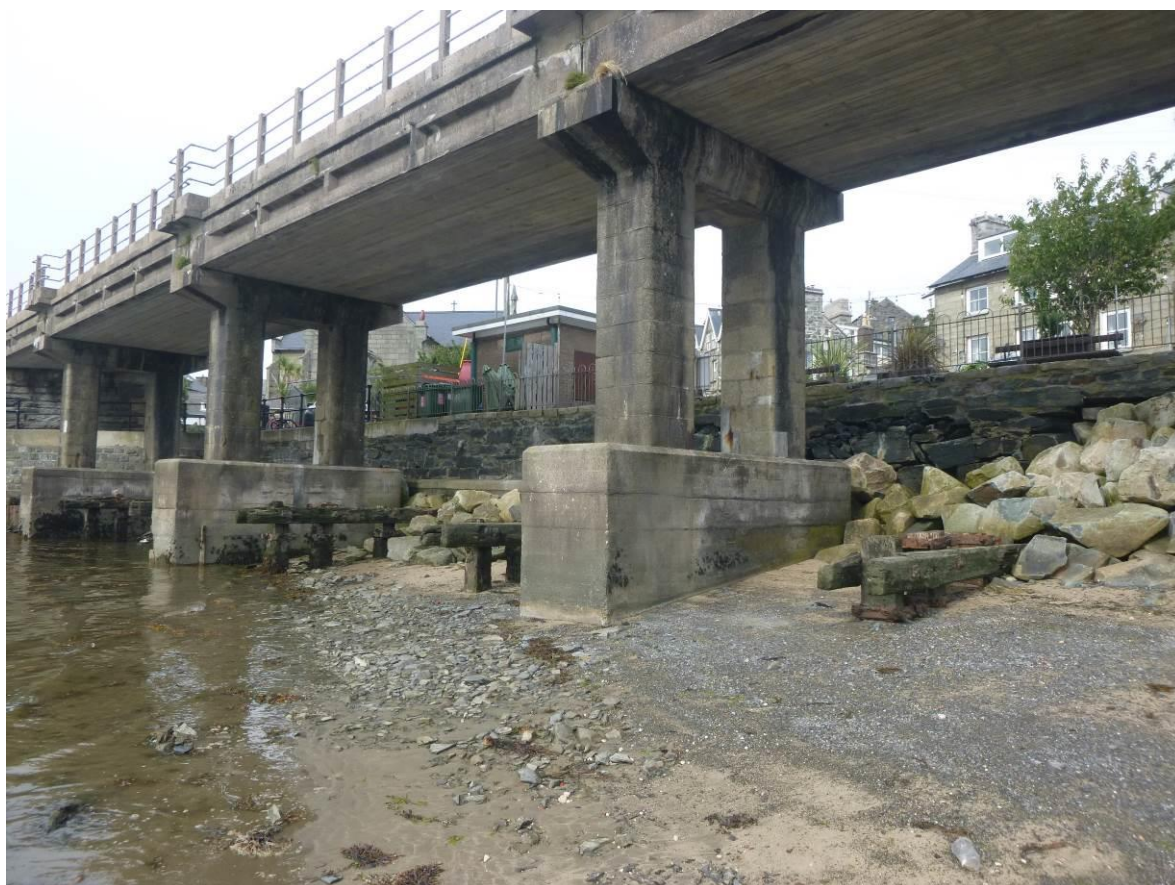
5. Western extent of frontage wall.
