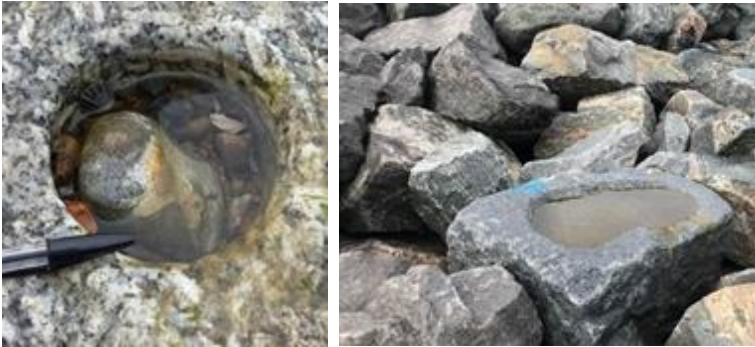
Figure 2. Examples of water retaining features in rock armour.
