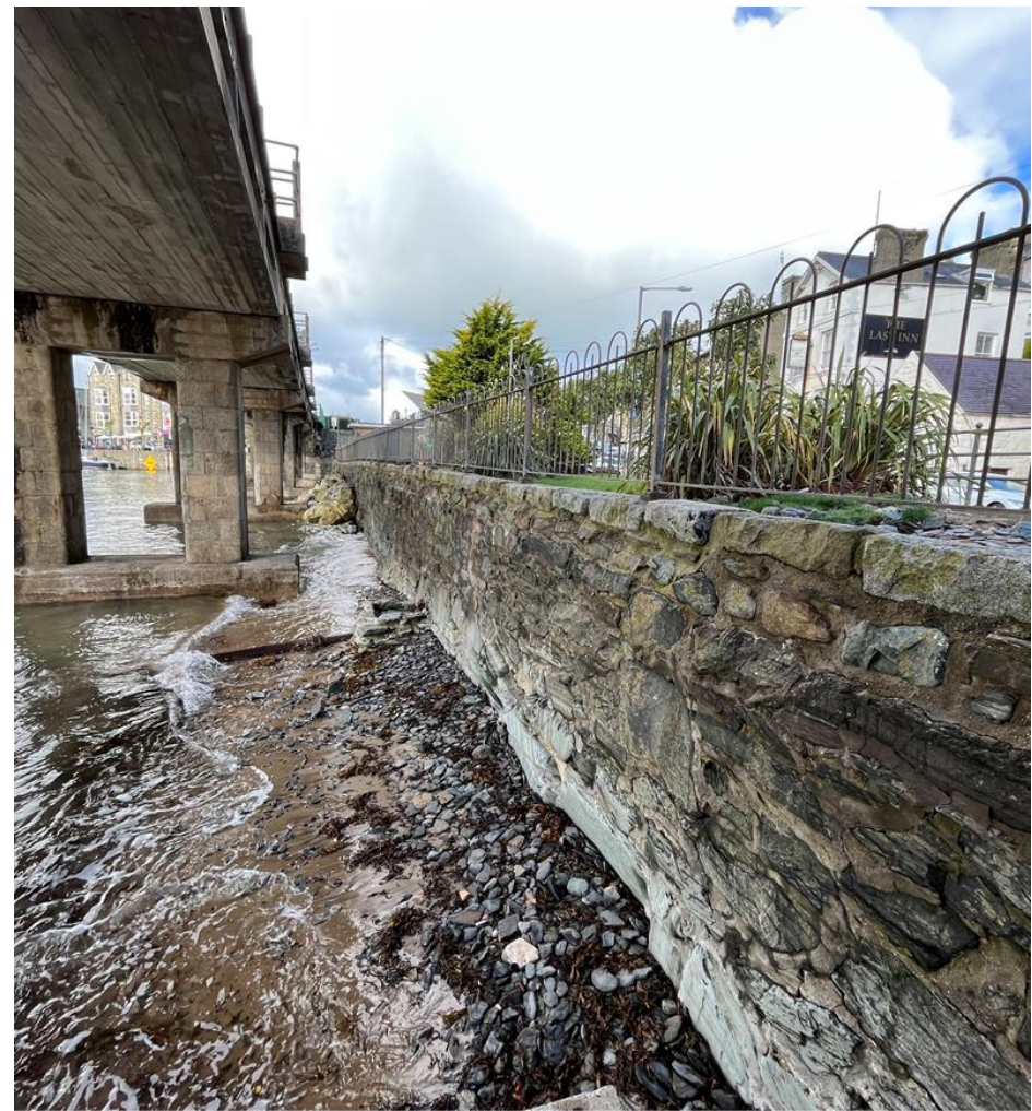
2. Looking west across the proposed works area.
