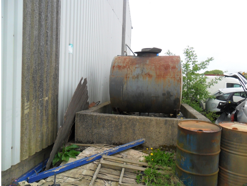
Photo of waste oil tank
