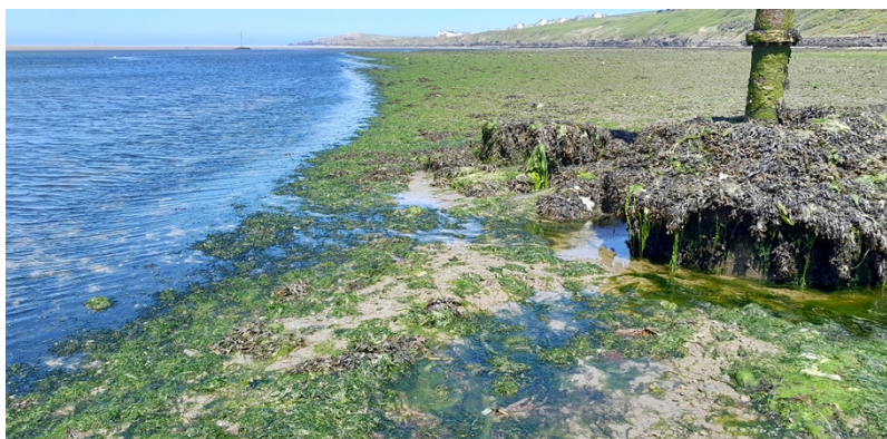
Photograph 1: Outfall at SN 15934 48626
