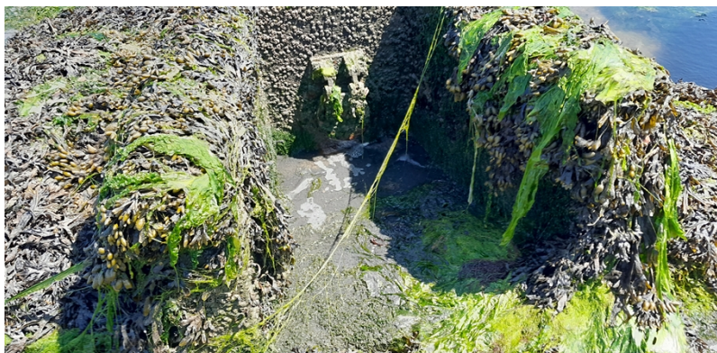
Photograph 2: Outfall at SN 15934 48626
