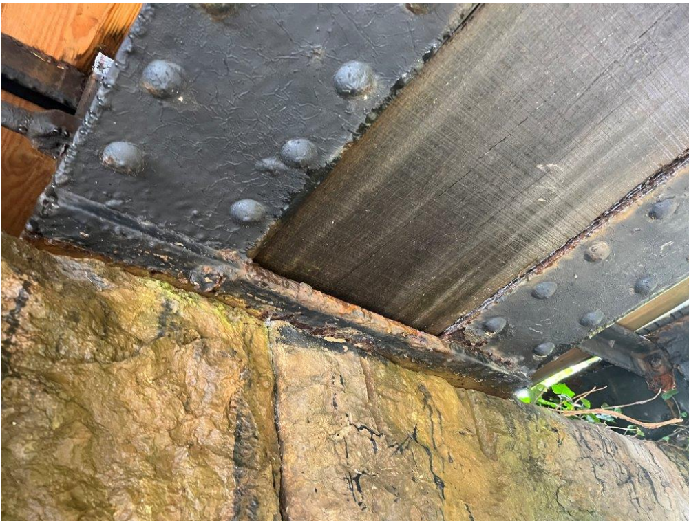
Photo 54: Typical view of bearing plate (02/08/22)
