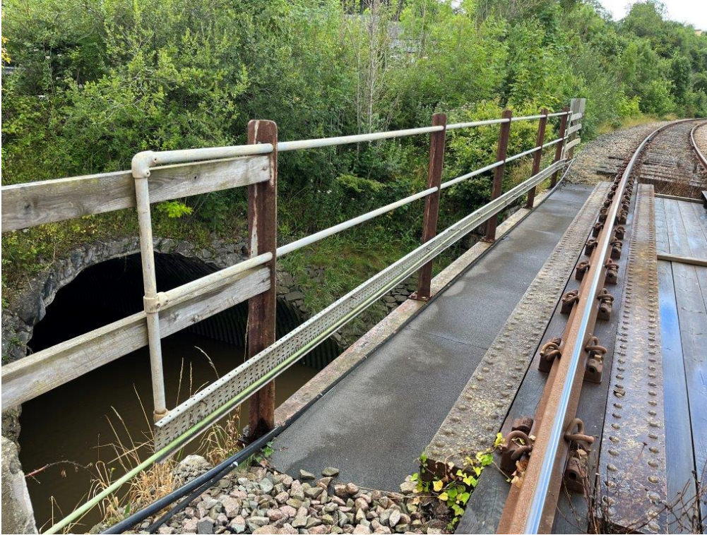
Photo 61: General view of Handrails (02/08/22)
