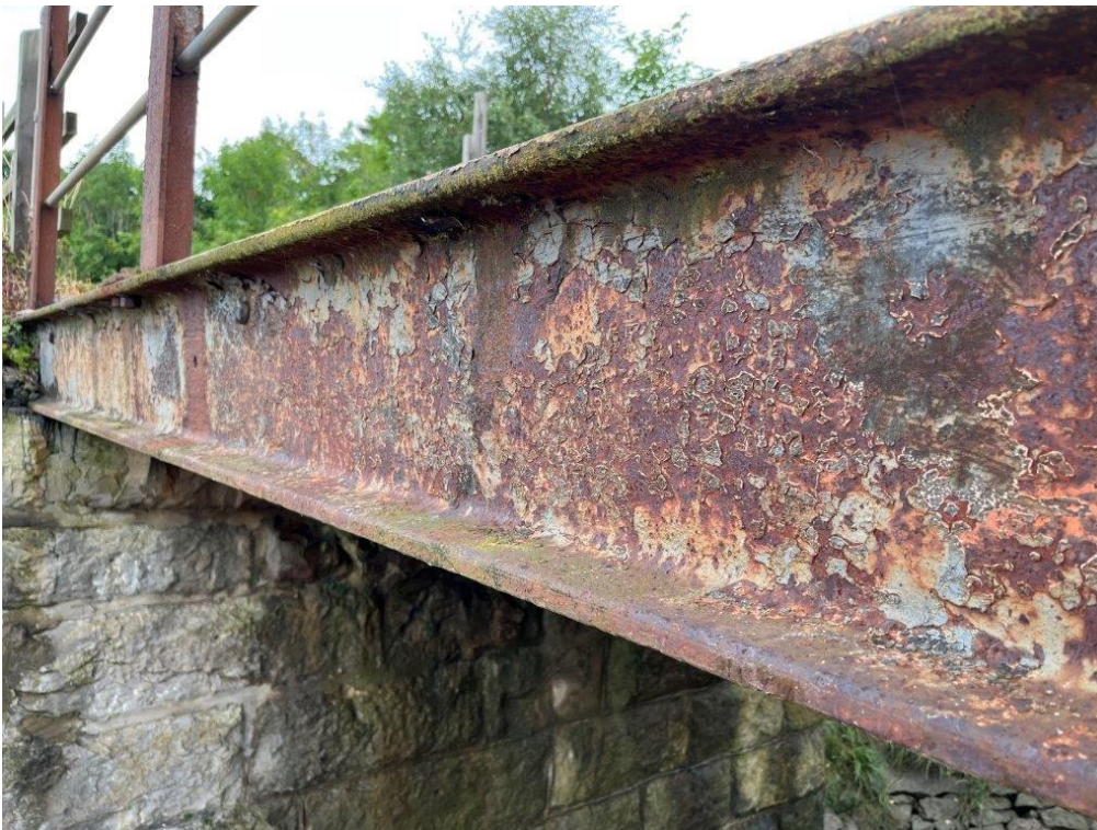
Photo 12: Upside Walkway Support Girder, mid-point towards LM (02/08/22)
