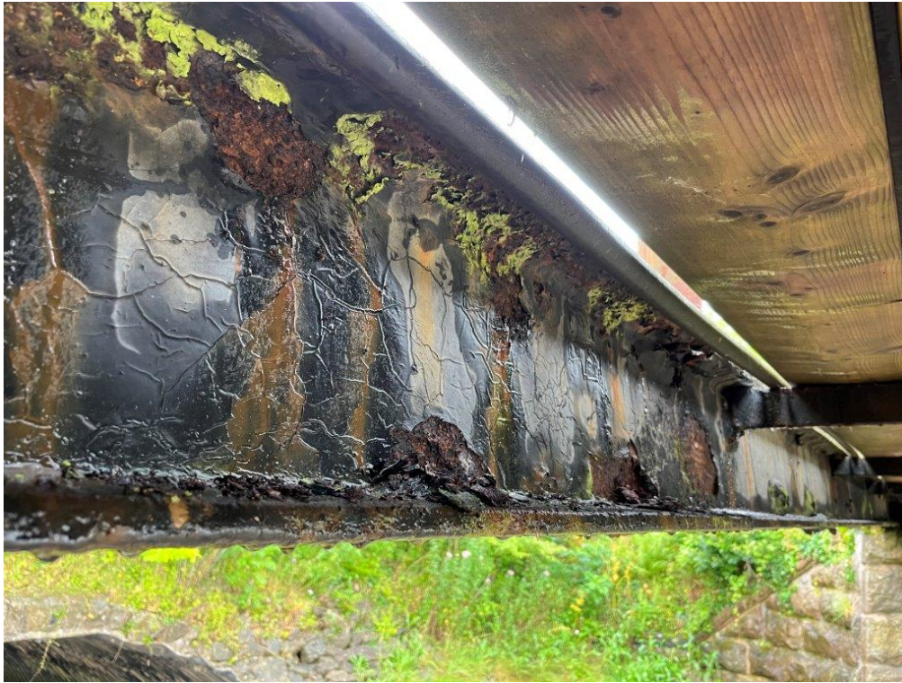
Photo 9: Inner face of DS Walkway Girder (02/08/22)
