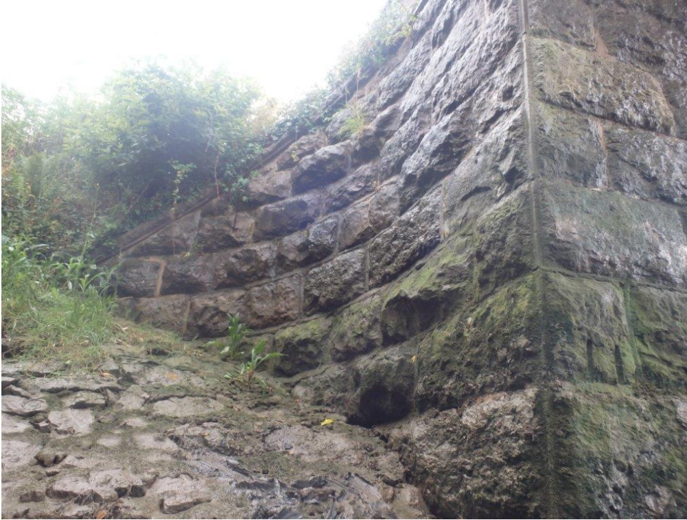
Photo 39: Downside High Mileage Wing Wall (02/08/22)
