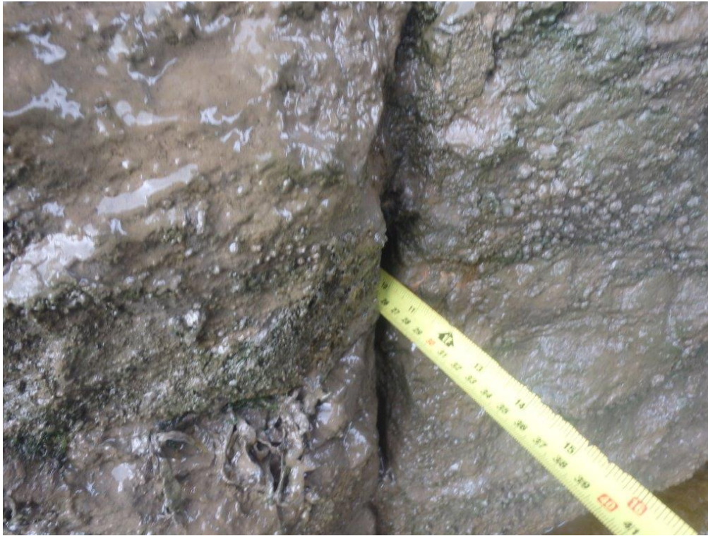
Photo 33: OJs to LM Abutment (02/08/22)
