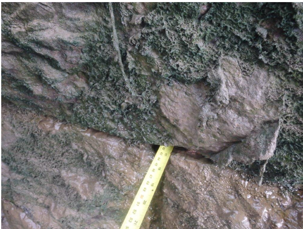
Photo 36: View of depth of OJs to HM Abutment (02/08/22)
