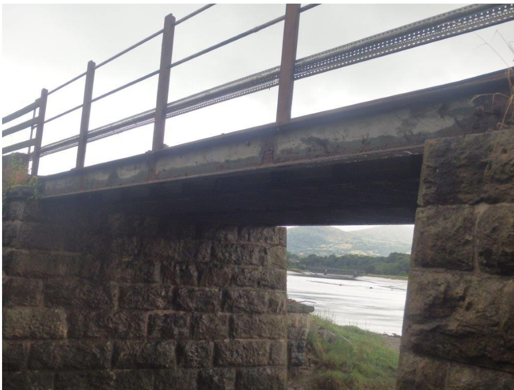
Photo 8: Downside Walkway Support Girder (02/08/22)
