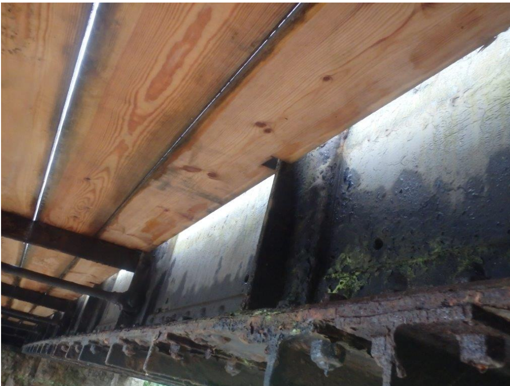
Photo 22: Upside Main Girder, DS Face (02/08/22)
