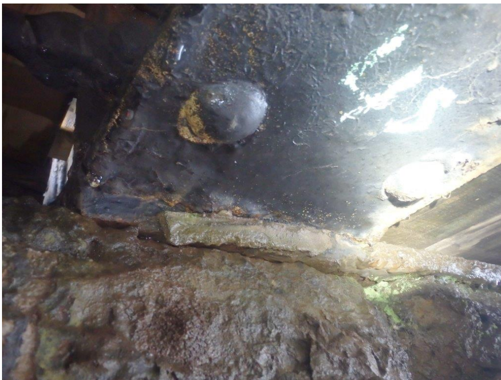
Photo 56: Mortar to outer edge of bearings (02/08/22)
