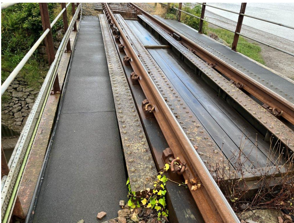
Photo 60: Typical view of Longitudinal Timbers (02/08/22)
