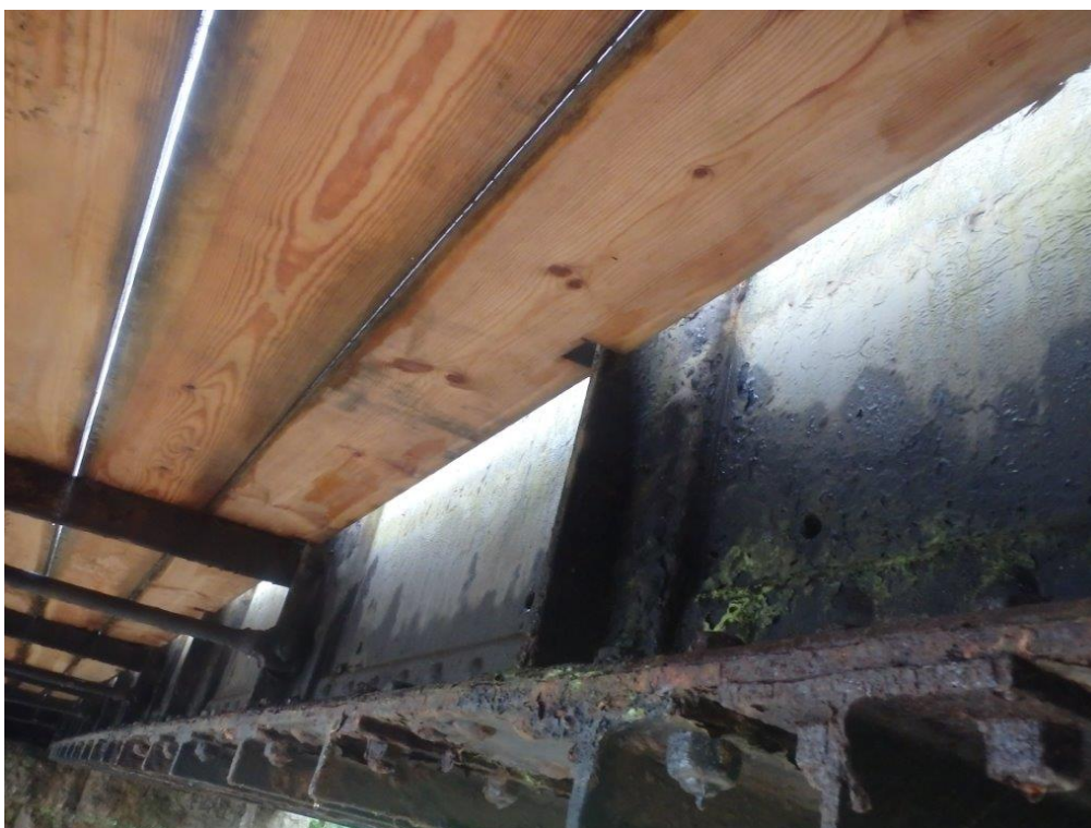
Photo 18: Downside Main Girder, US Face (02/08/22)
