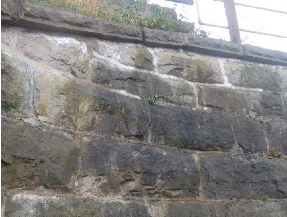
Photo 51: Repointing works to upper reaches, US LM Wing Wall (02/08/22)
