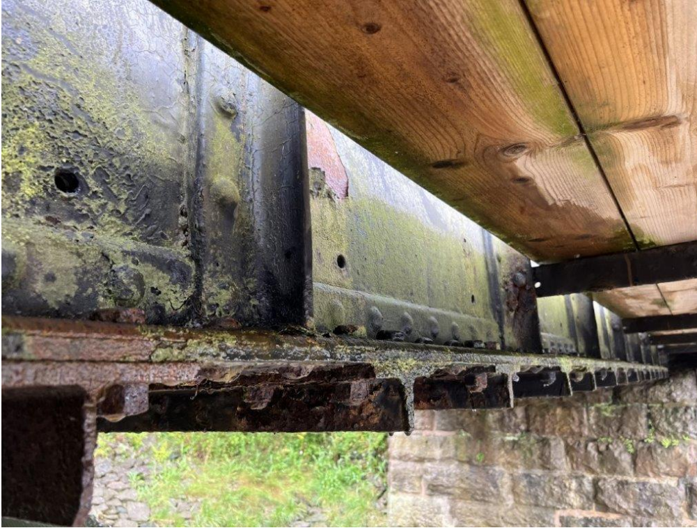
Photo 21: Upside Main Girder, US Face (02/08/22)
