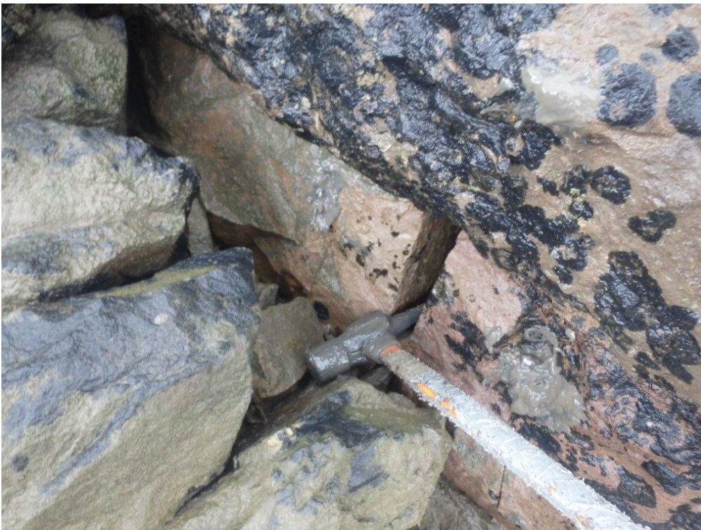
Photo 50: OJs to US LM Wing Wall (02/08/22)
