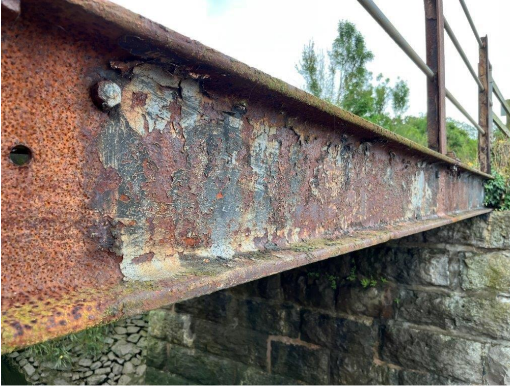
Photo 11: Upside Walkway Support Girder, mid-point towards HM (02/08/22)
