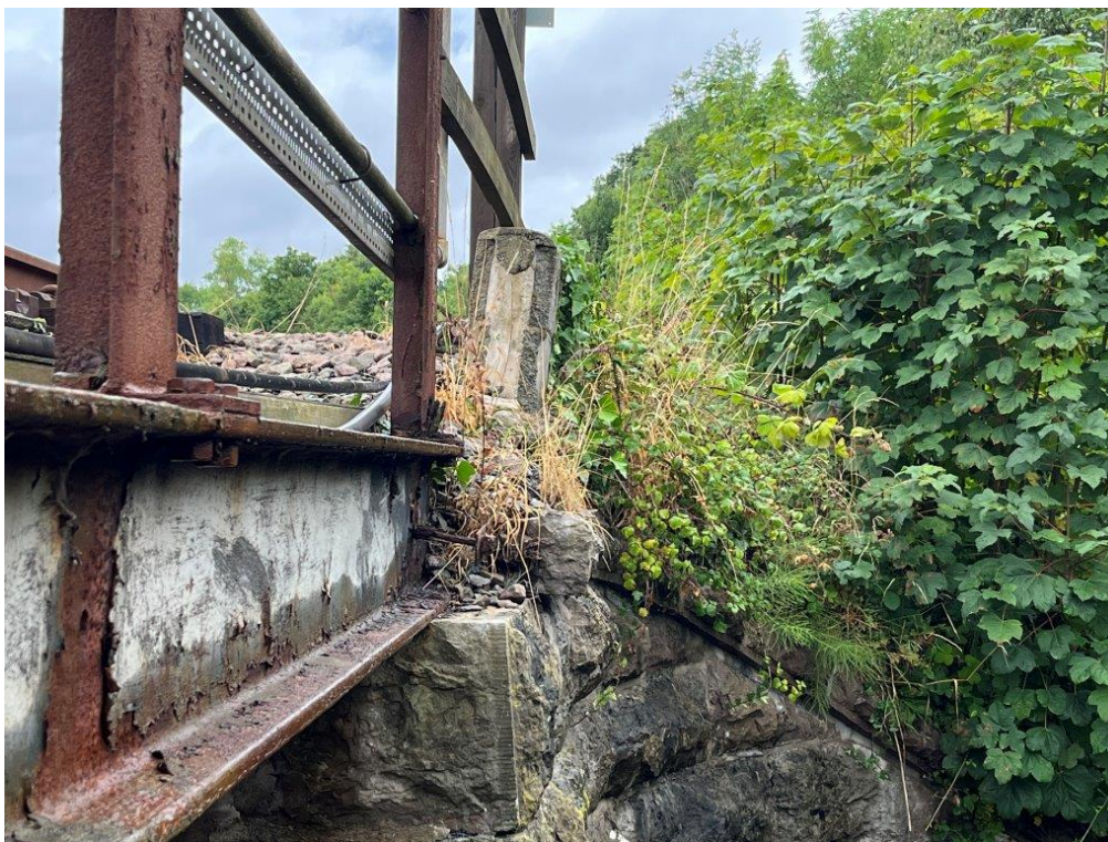
Photo 59: Lean to DS LM Ballast Wall (02/08/22)
