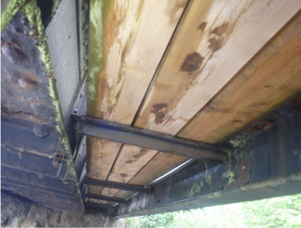
Photo 27: Downside Walkway / DCK (02/08/22)
