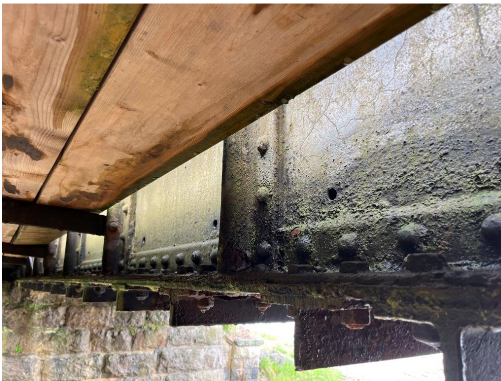
Photo 17: Downside Main Girder, DS Face (02/08/22)
