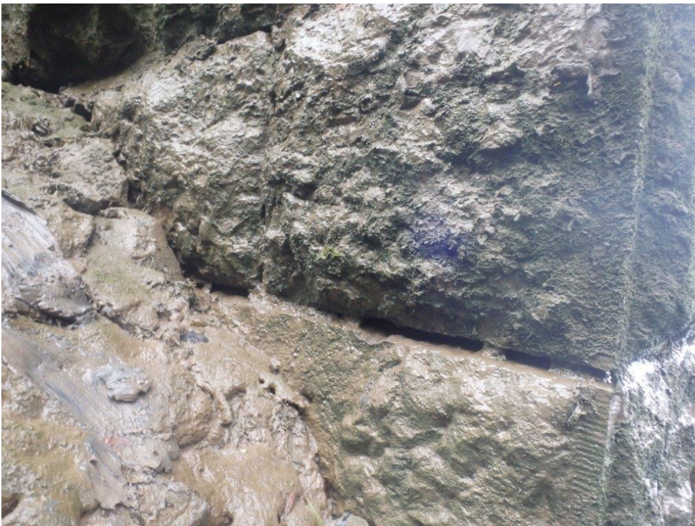
Photo 40: OJs to DS HM Wing Wall (02/08/22)
