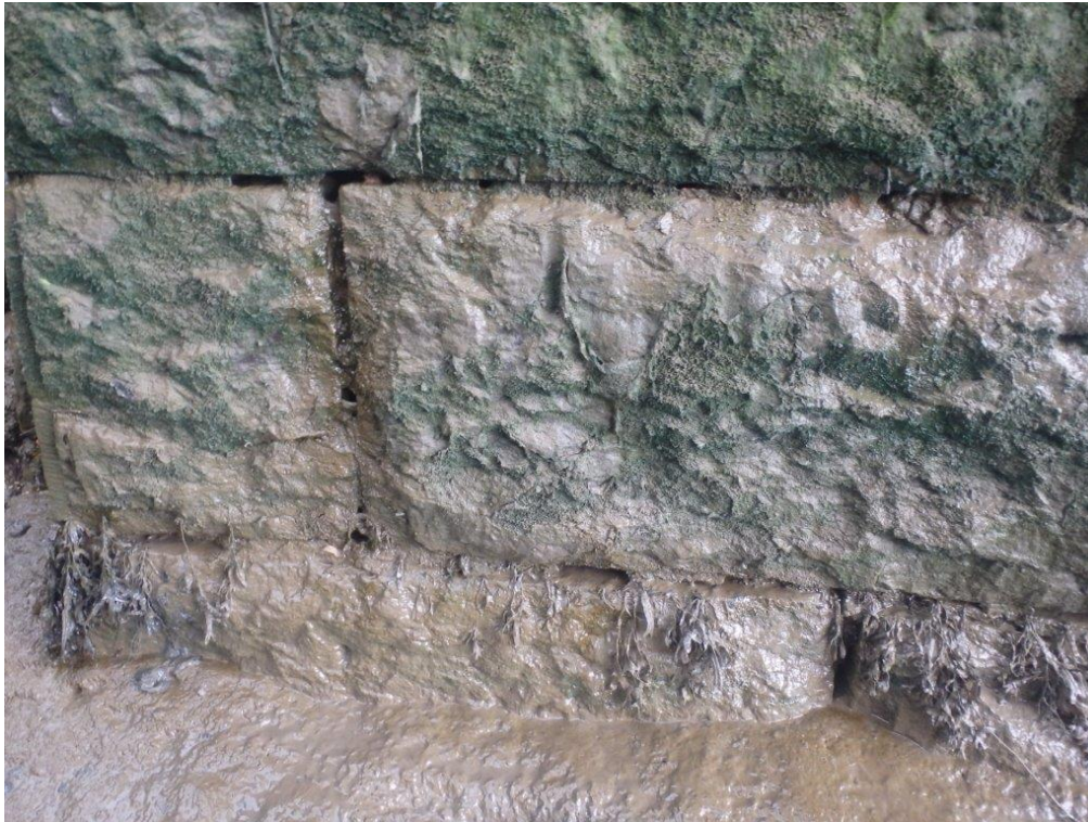
Photo 35: OJs to lower reaches of HM Abutment (02/08/22)
