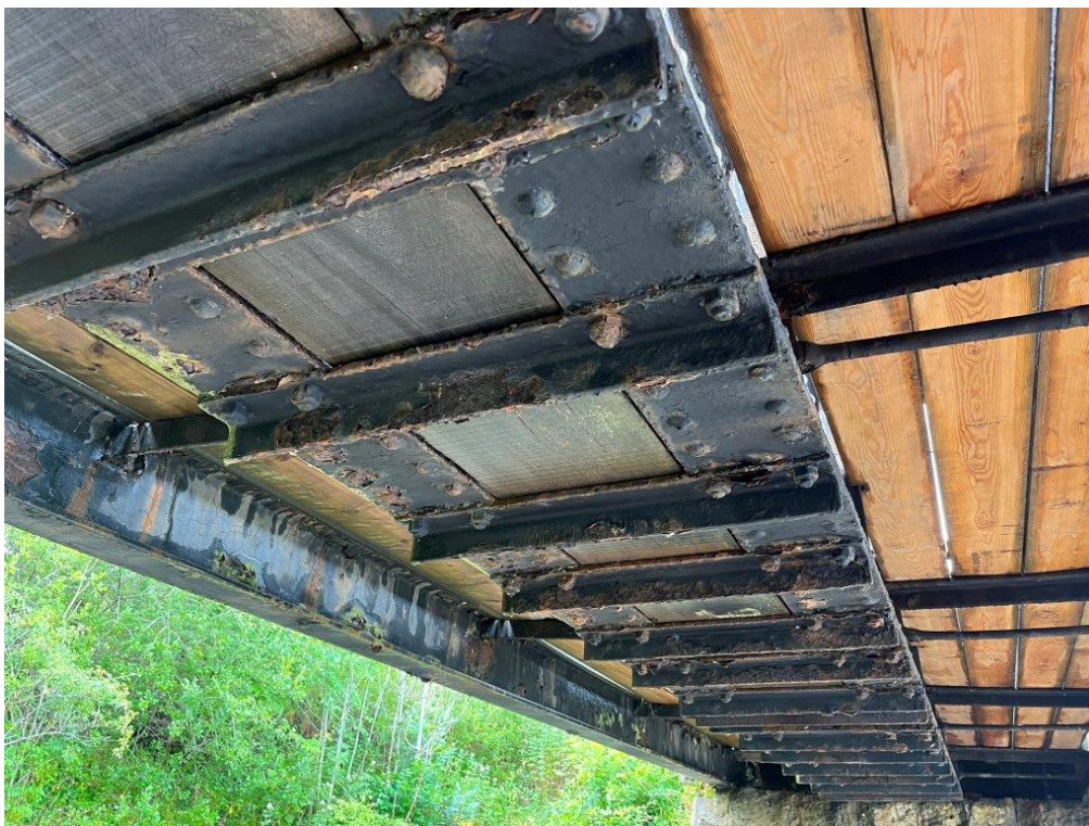
Photo 19: Soffit of DS Main Girder (02/08/22)
