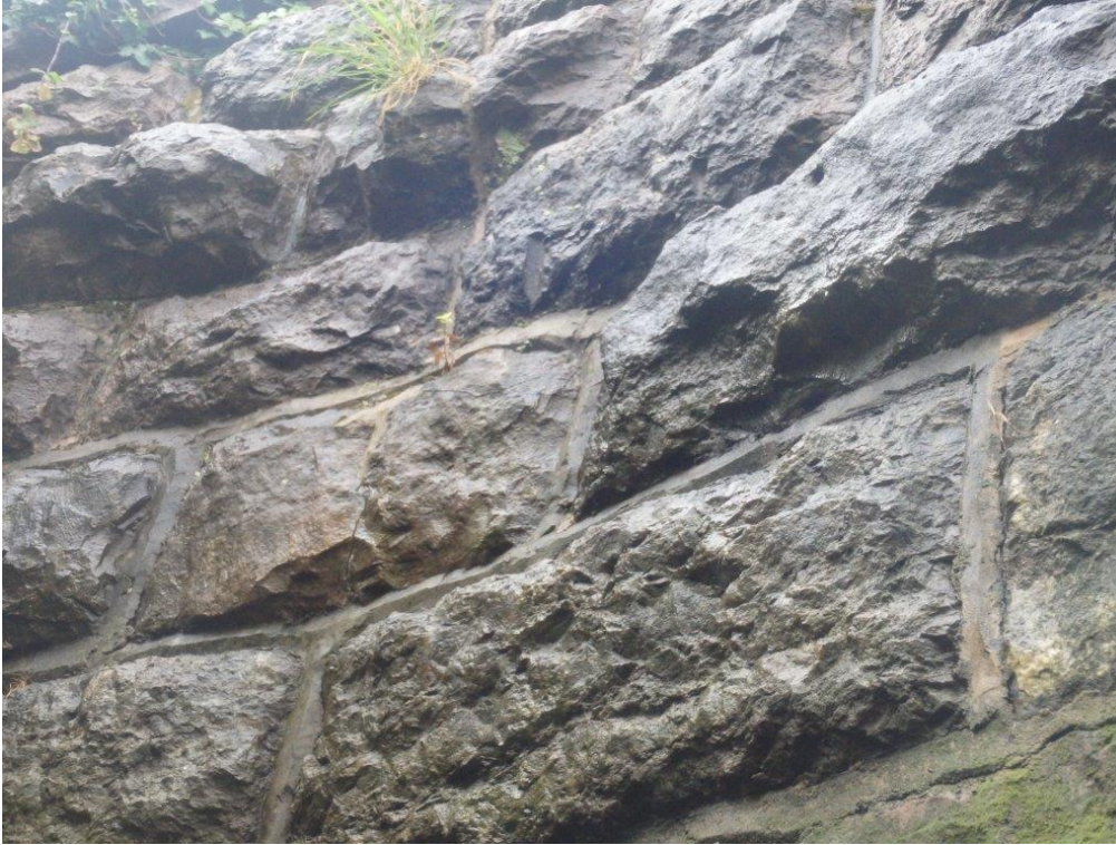
Photo 41: View of split stones, DS HM Wing Wall (02/08/22)
