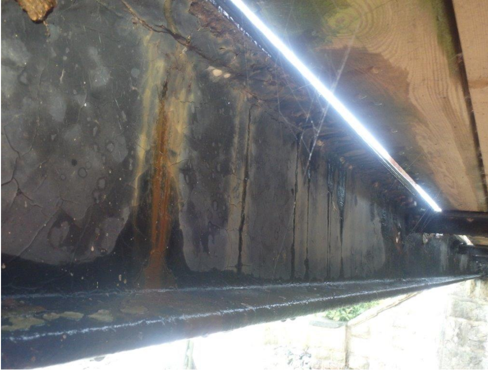
Photo 13: Inner Face of US Walkway Support Girder (02/08/22)
