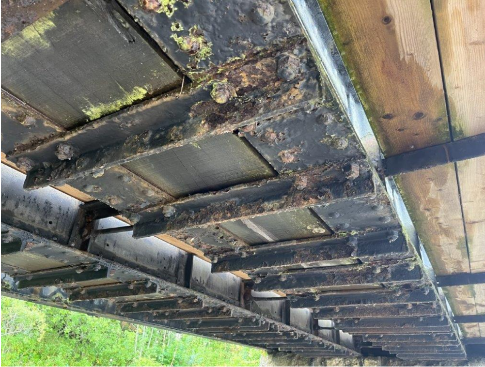
Photo 23: Soffit of US Main Girder (02/08/22)
