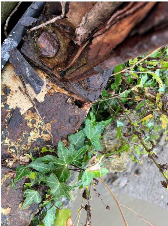
Photo 15: LOS to US Walkway Support Girder (02/08/22)
