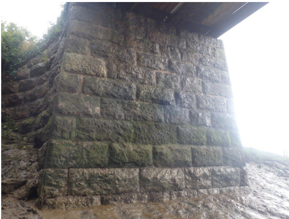
Photo 34: High Mileage Abutment (02/08/22)
