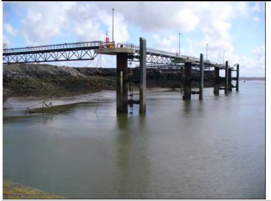
Figure 2.4 Breakwater and Catwalk Pier
