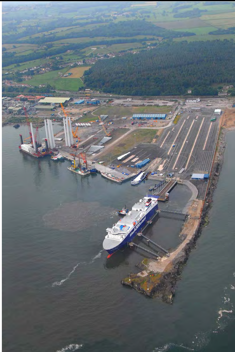
Figure 2.1 Port of Mostyn Showing the Ro-Ro Facility in use
