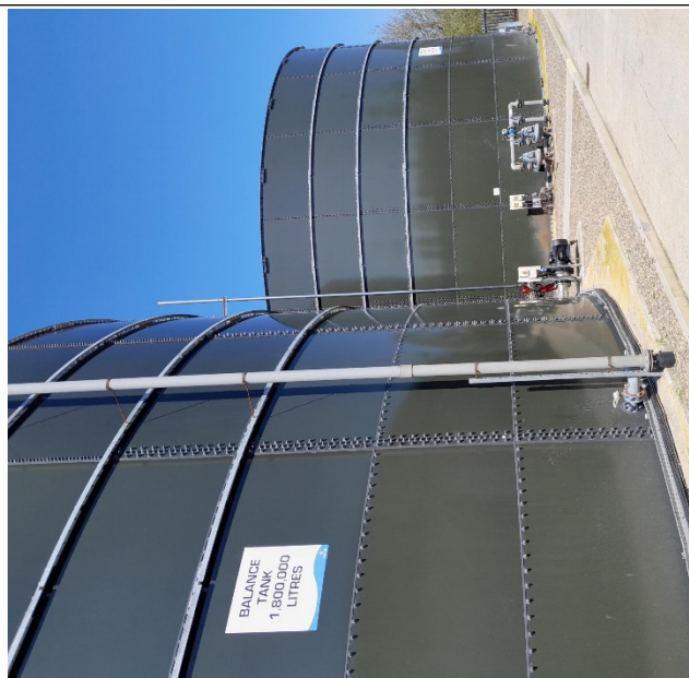
Pics 8 & 9; Permastore balance tanks on the effluent treatment plant. No secondary containment. Annual NDT structural integrity tests are carried out. Site relies upon tertiary collection of spills but does not account for a major collapse.
