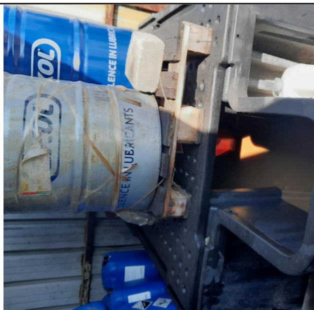
Pic 5. Temporary secondary containment used in the oil store. Bund should be routinely emptied to ensure space is left in the bund in the event of a failure.
