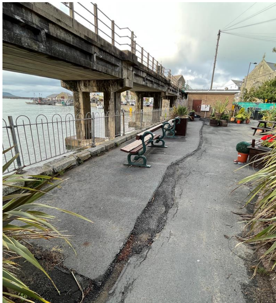
4. Viaduct Gardens area, north of the frontage wall.
