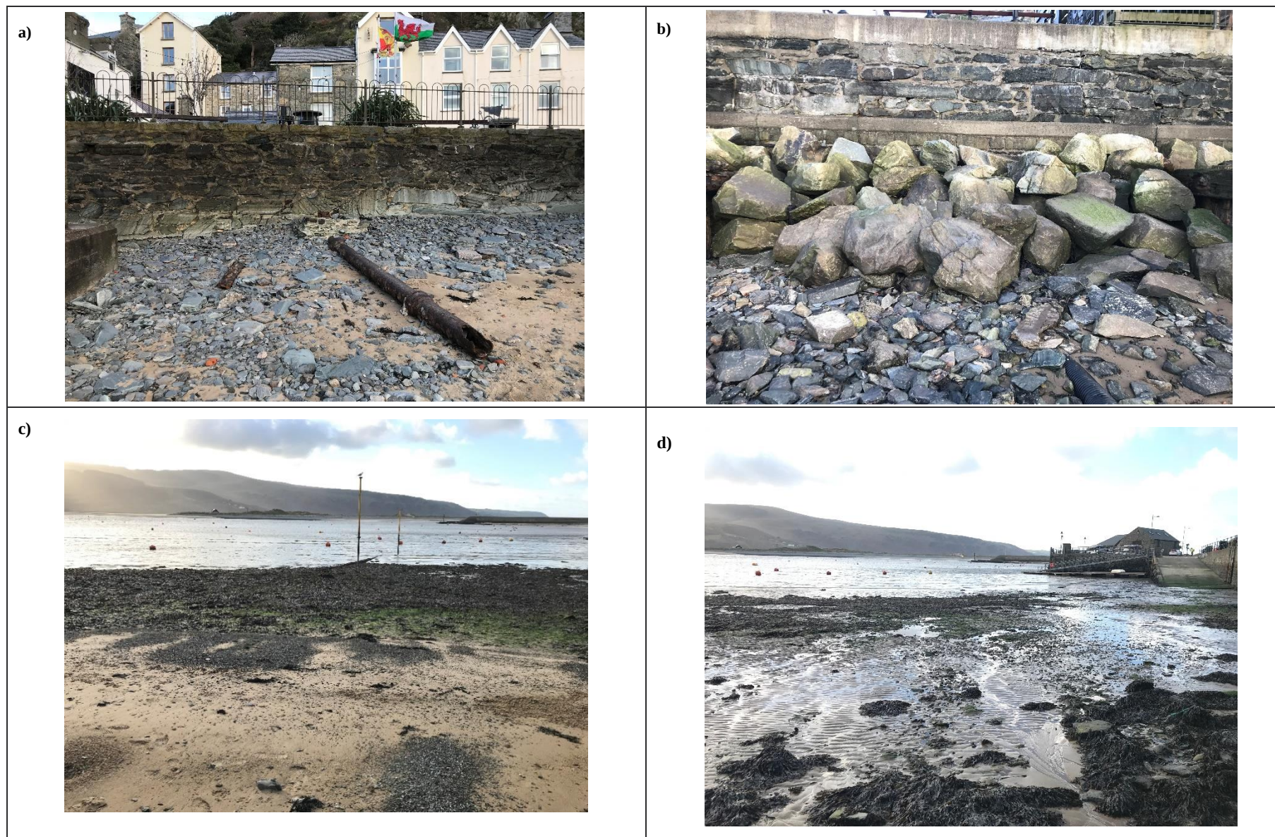
Figure 3: Top Left: Frontage 1 seawall; view north. Top right; Frontage 1 seawall and rock armour; view north. Bottom Left: Frontage 1 intertidal area, view south. Bottom right: Frontage 1 intertidal area, view south.
