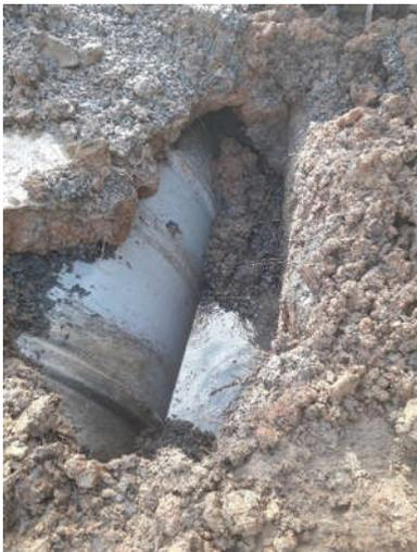
**Photo 14:** TP-3 and TP-4 were advanced next to the septic tank. Groundwater entered the excavations between 1.5 – 2.0 m.
