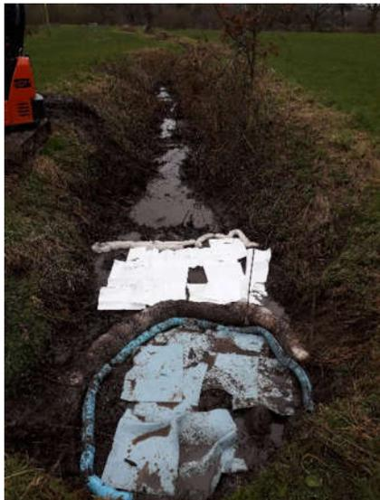
**Photo 9:** Absorbent booms and mats were deployed next to the brook opening.
