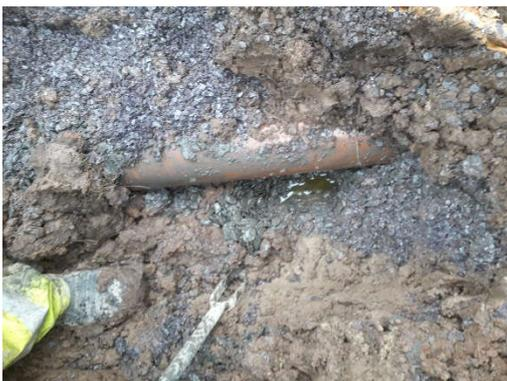
**Photo 12:** The foul pipe was exposed in TP-1 and neat product was identified. Gravels around the pipe were significantly contaminated.
