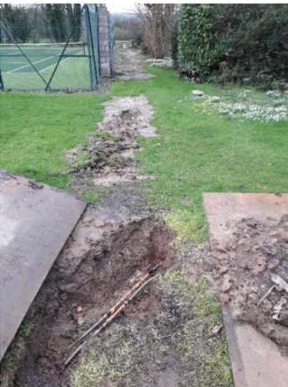
**Photo 3:** Spill origin excavation exposing damaged feedline.
