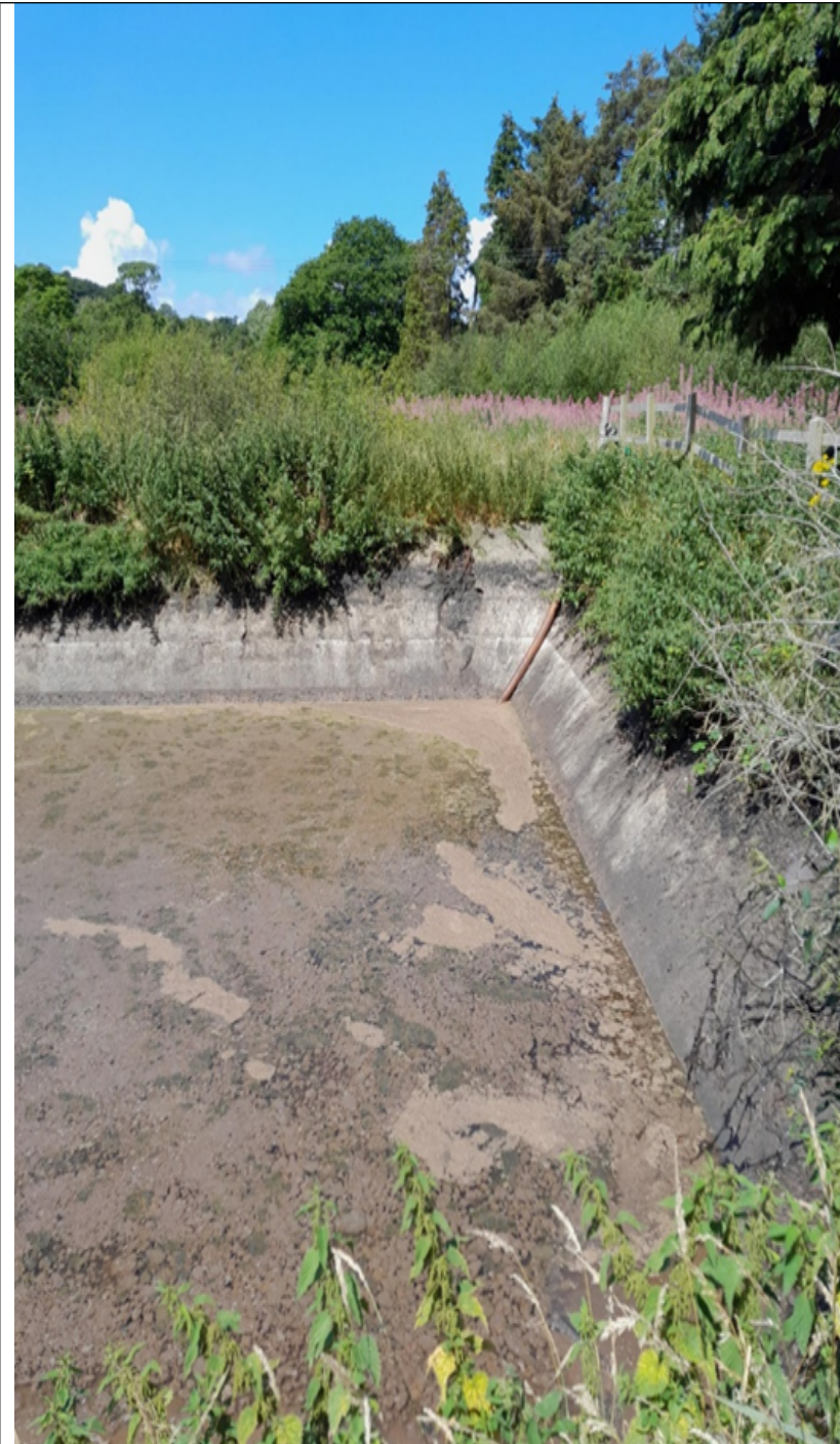
Photo 4: sludge settlement lagoon
