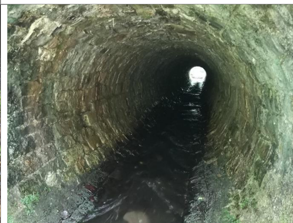
Figure 7-6. Culverted section of the watercourse beneath the canal. A vertical fall was visible at the upstream end of the culvert.
