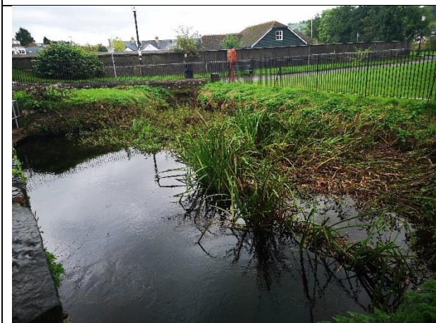
Figure 3-5. The settling pond between the river frontage intake and the culvert supplying the canal.
