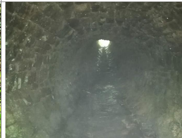
Figure 6-6. Culverted section of the watercourse beneath the canal.
