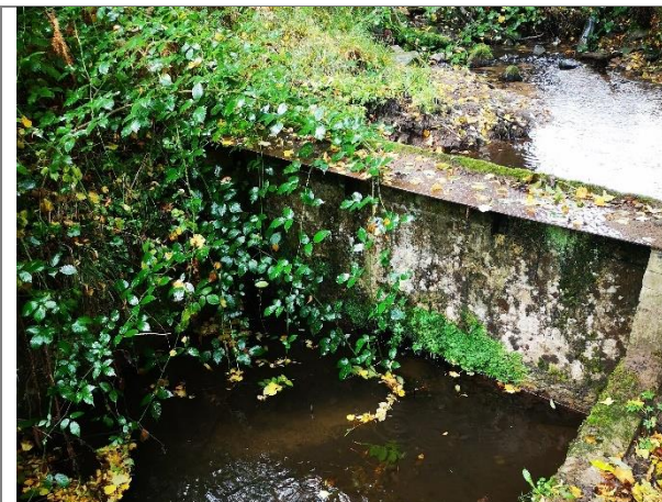
Figure 7-3. Downstream face of the submerged orifice supplying the feeder channel.
