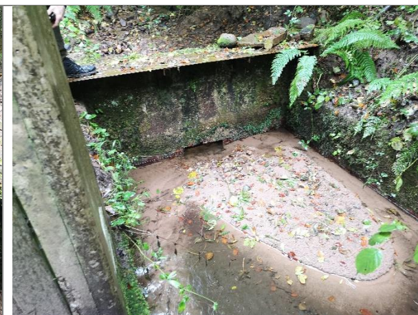
Figure 6-3. Downstream face of the submerged orifice supplying the feeder channel.
