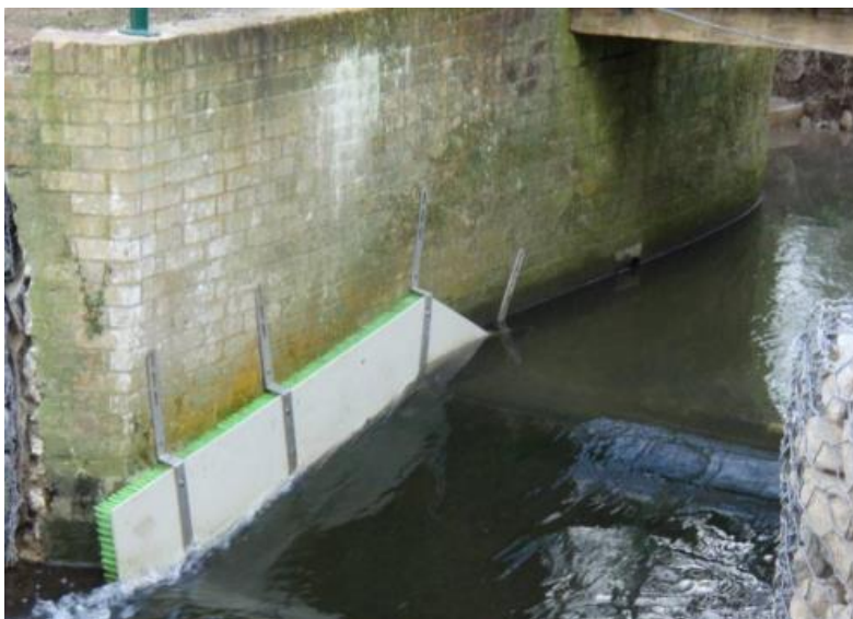
Figure 5-8. An example of a vertical eel brush pass fixed to a weir wing wall.
