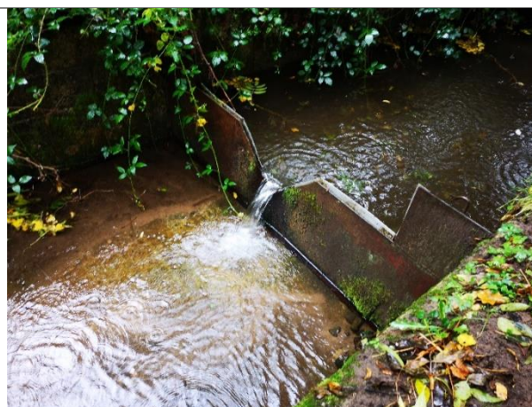
Figure 7-2. Penstock on the upstream face of the submerged orifice supplying the feeder channel.
