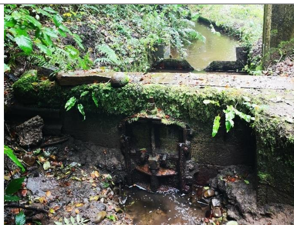
Figure 6-2. Penstock on the upstream face of the submerged orifice supplying the feeder channel.
