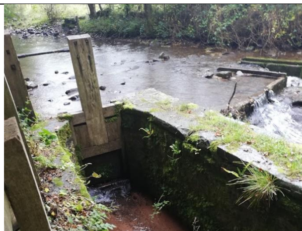
Figure 4-2. The Cwm Crawnnon sluice gate and upstream end of the leat channel.
