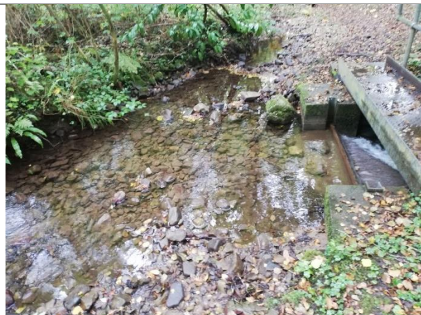
Figure 5-2. The weir board structure at bifurcation 1 on the Nant Onnau Fach. Water supplying the canal flows to the top of the image.
