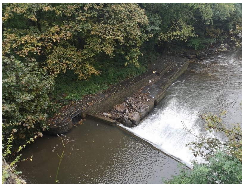
Figure 10-1. The Larinier super-active baffle fish pass on the true left bank of the Pontymoile weir, 50 m downstream of the proposed abstraction location.
