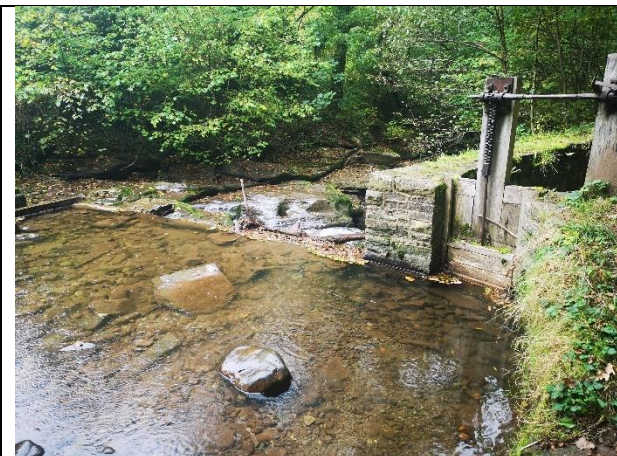
Figure 4-1. The location of the existing Cwm Crawnnon intake/sluice gate relative to the weir crest.
