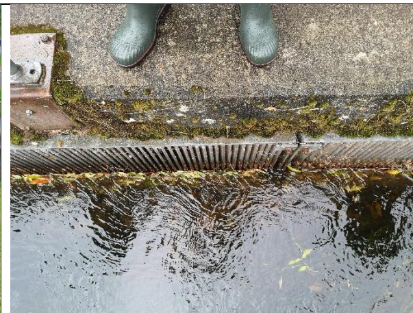
Figure 3-4. Existing 10 mm rectangular profile bar screening at the river frontage.
