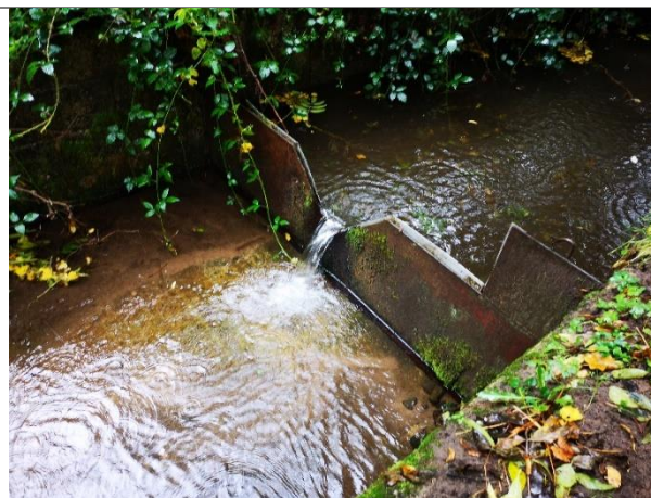
Figure 7-5. V-notch weir on the abstraction (feeder) channel.
