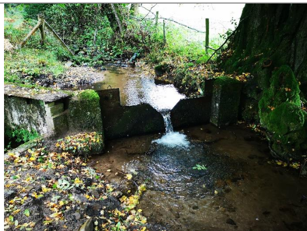
Figure 7-1. V-notch weir on the main river channel at Ochram Turn.
