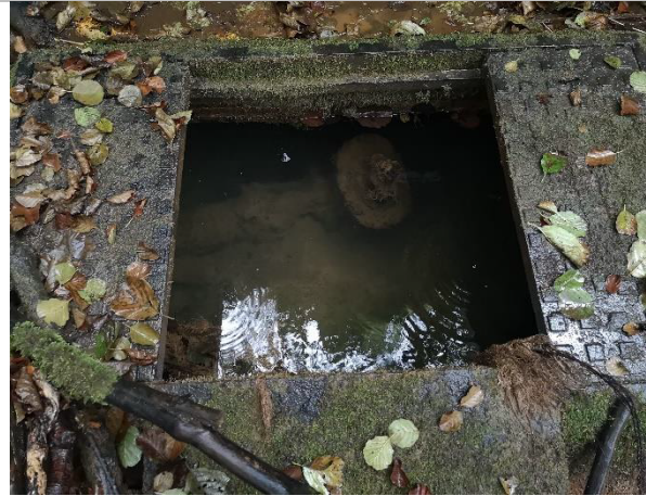
Figure 9-2. Manhole cover on the top of the Trosnant Spring intake structure.
