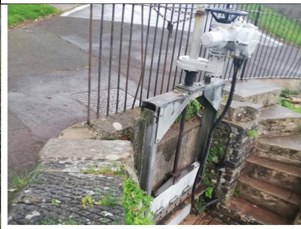
Figure 3-7. Penstock controlling flow from the settling pond into the culvert, ultimately supplying the canal.
