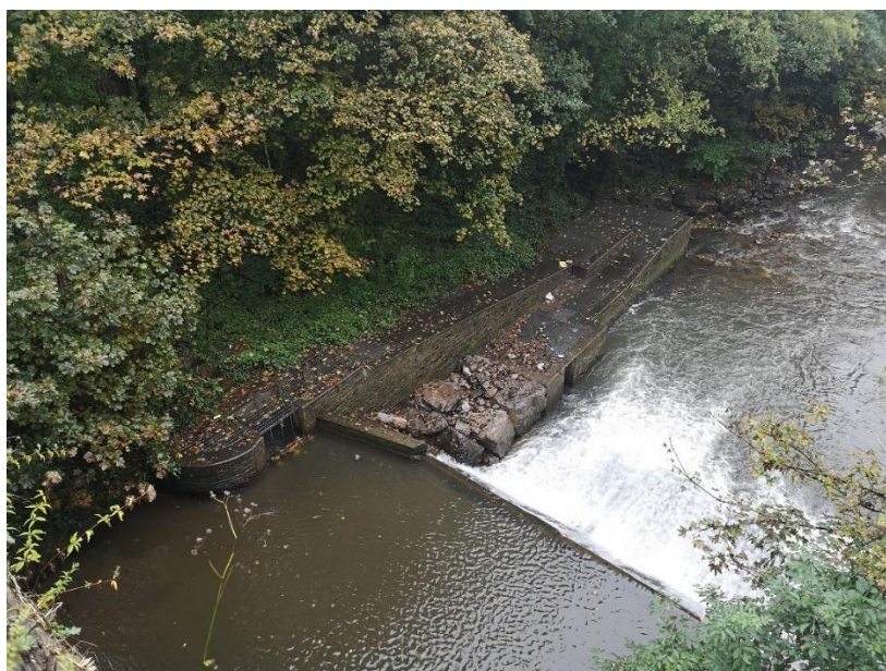
Figure 10-1. The Larinier super-active baffle fish pass on the true left bank of the Pontymoile weir, 50 m downstream of the proposed abstraction location.
