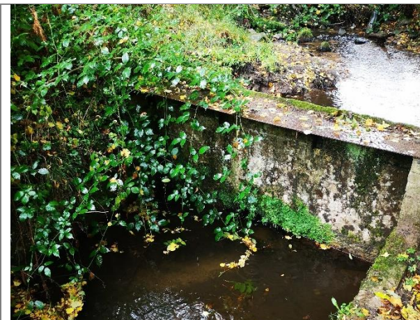
Figure 7-3. Downstream face of the submerged orifice supplying the feeder channel.
