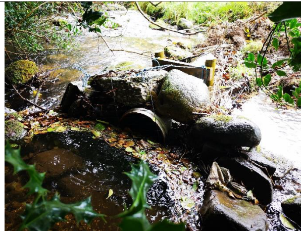
Figure 8-2. Close up of the metal screen on the pipe opening.
