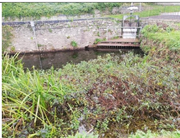
Figure 3-6. Coarse debris screening in front of the culvert penstock.
