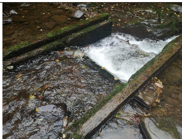
Figure 4-5. The two pools in the fish pass easement structure upstream of the crest at Cwm Crawnnon.
