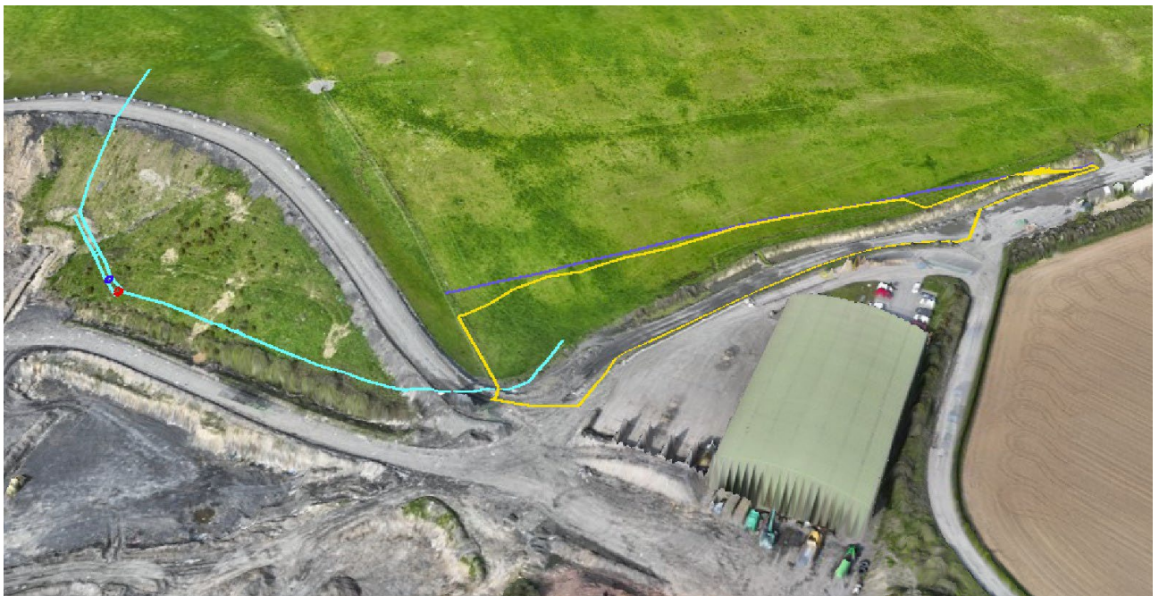
Figure 1-2 Cell 13 Works Area
