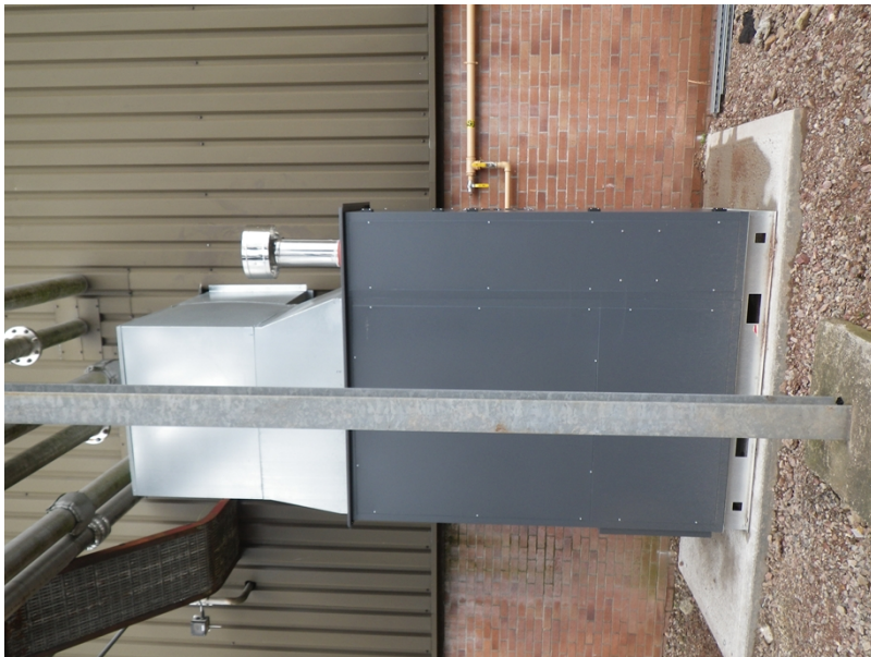
Photo 10: Small gas generated heater at the liming pits
