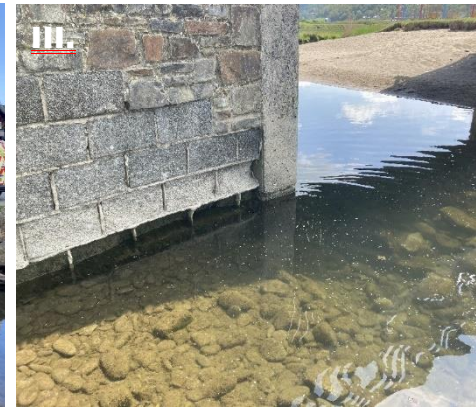
I. View of east/upstream parapet with the upstream line of scour protection boulders. II. As I, but from the southern embankment, showing the small gap between existing scour protection boulders and the east parapet. III. View of scour on west/downstream parapet. IV. As III, but from southern embankment – scour protection boulders of former carpark also visible.
