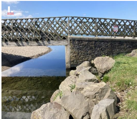
I. View of east/upstream parapet with the upstream line of scour protection boulders. II. As I, but from the southern embankment, showing the small gap between existing scour protection boulders and the east parapet. III. View of scour on west/downstream parapet. IV. As III, but from southern embankment – scour protection boulders of former carpark also visible.
