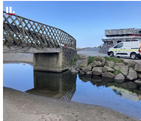
I. View of east/upstream parapet with the upstream line of scour protection boulders. II. As I, but from the southern embankment, showing the small gap between existing scour protection boulders and the east parapet. III. View of scour on west/downstream parapet. IV. As III, but from southern embankment – scour protection boulders of former carpark also visible.
