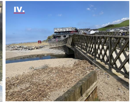
I. View of east/upstream parapet with the upstream line of scour protection boulders. II. As I, but from the southern embankment, showing the small gap between existing scour protection boulders and the east parapet. III. View of scour on west/downstream parapet. IV. As III, but from southern embankment – scour protection boulders of former carpark also visible.
