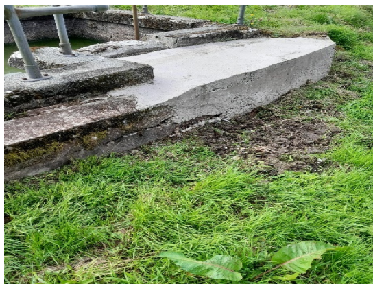
Image 2 – Repairs to primary tank.
