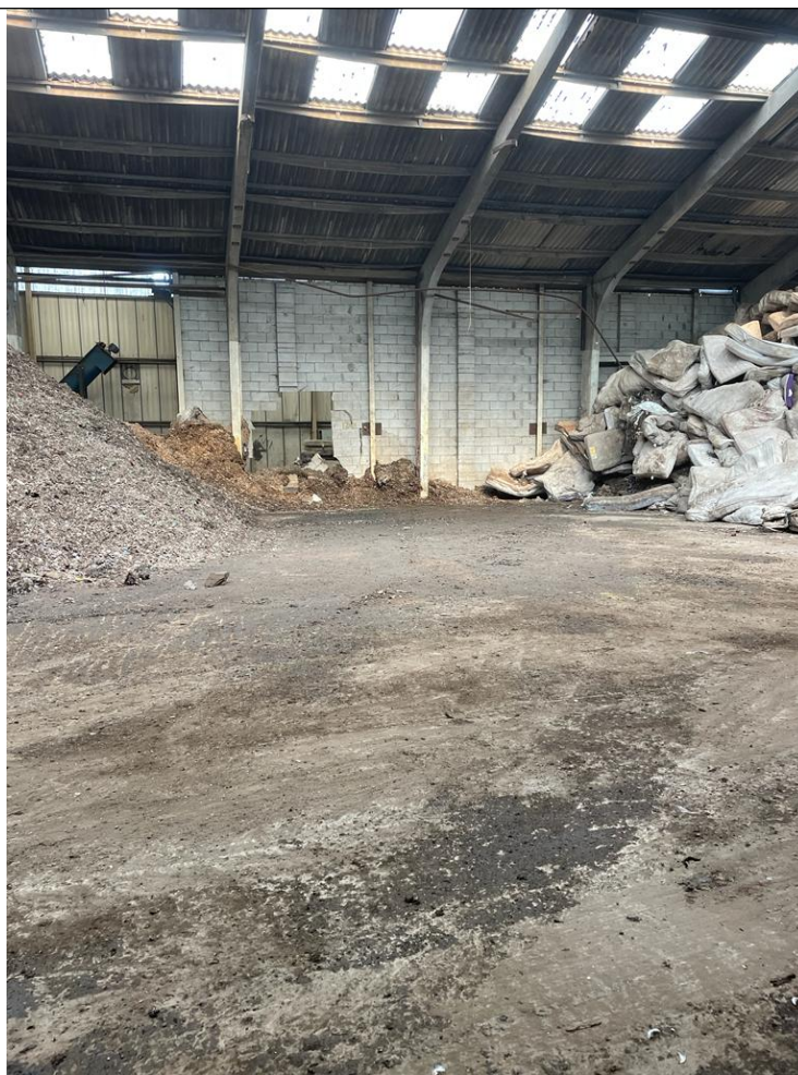
Photo 3 – Mr. THOMAS sent a photo showing improved distances between stockpiles
