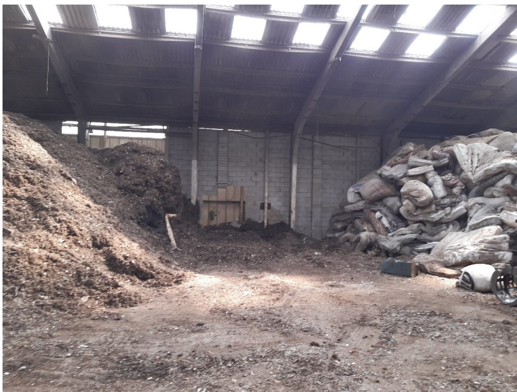
Photo 1 – distances between stockpiles of combustible material (RDF on the left)
