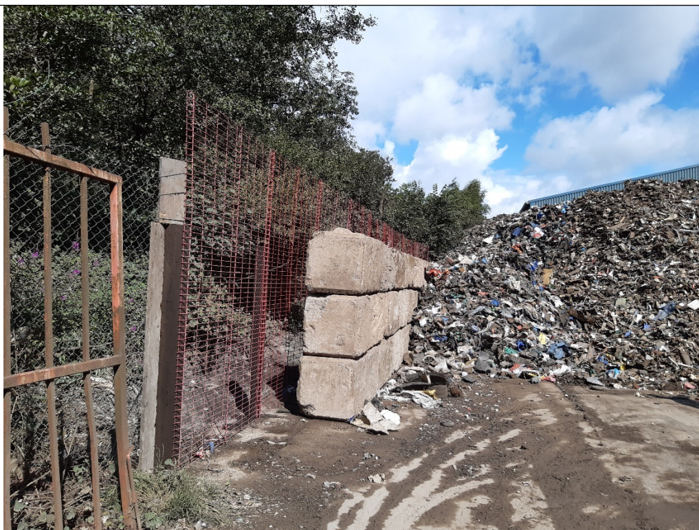
Photo 6 – newly installed security fencing in the yard between units 5 and 6
