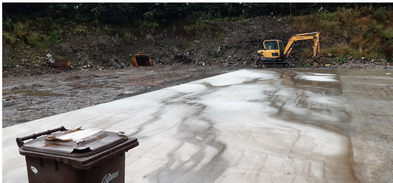
Photo 4 - Flooring infrastructure improvements at Bryn Recycling Ltd
