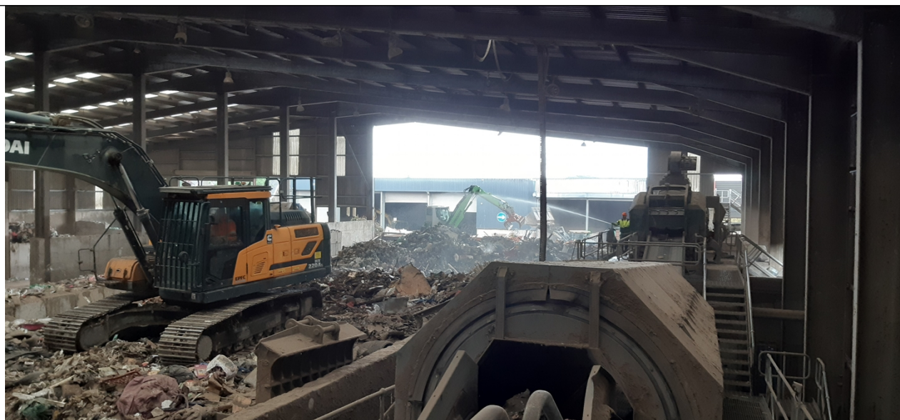
Photo 7 - Stockpile of waste(s) within waste transfer station building and dust suppression techniques being undertaken (background off centre (right))
