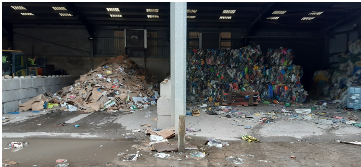
Photo 1 - View inside waste transfer station building
