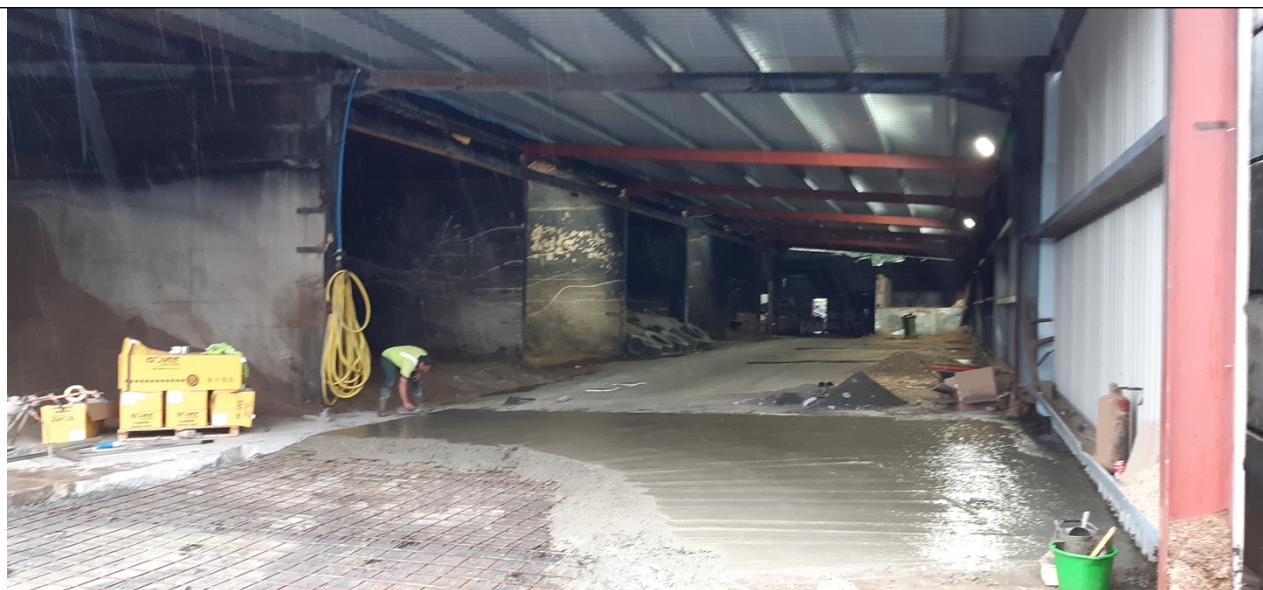
Photo 9 - Drying sheds area with infrastructure improvements taking place
