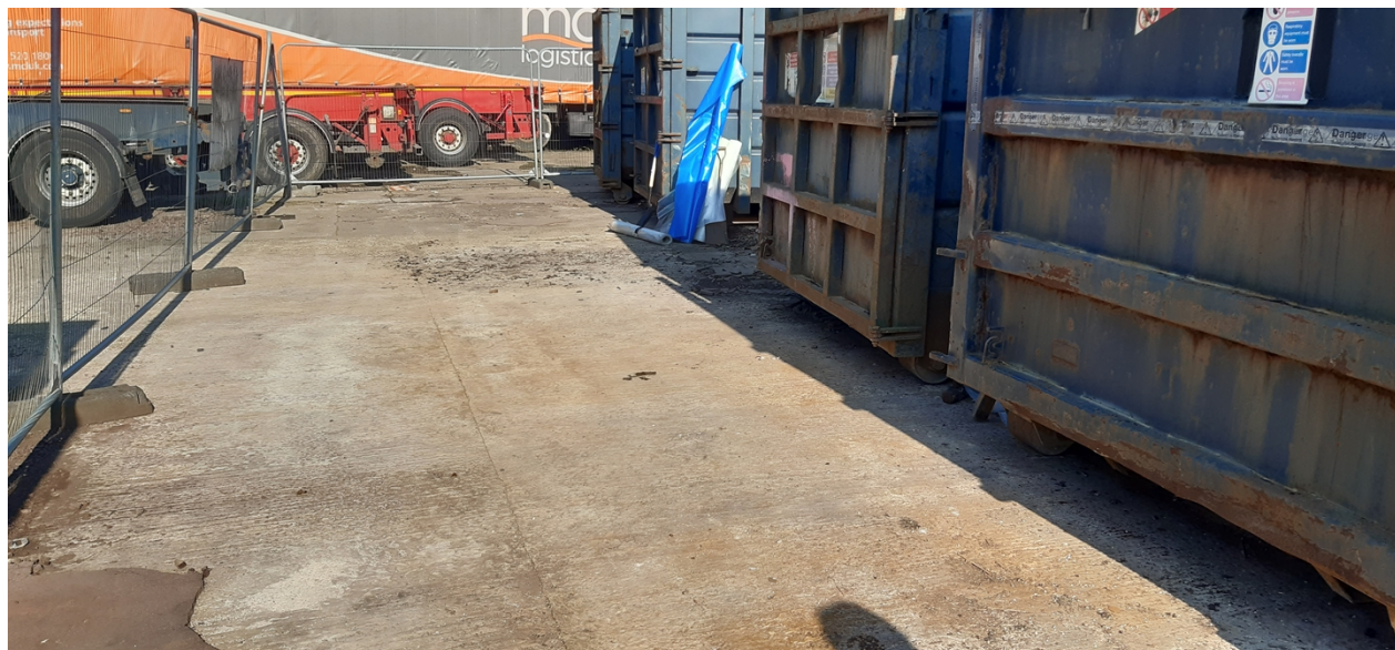
Photo 2 - Windsor Waste Management Ltd Asbestos Storage Area Infrastructure
