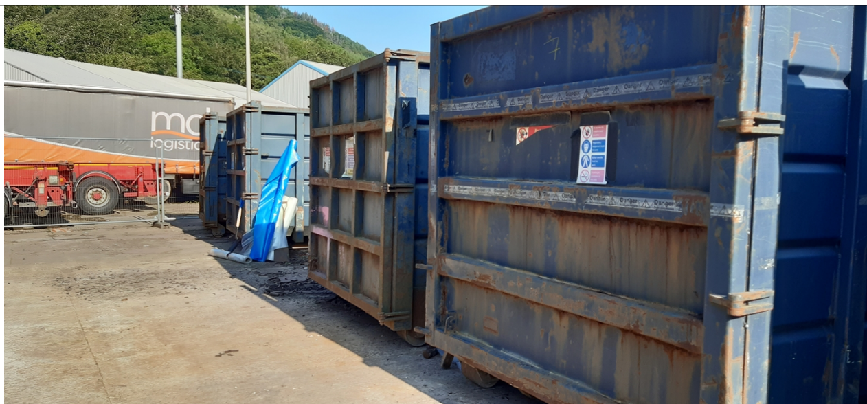
Photo 3 - Windsor Waste Management Ltd Asbestos Storage Area Secured Containers
