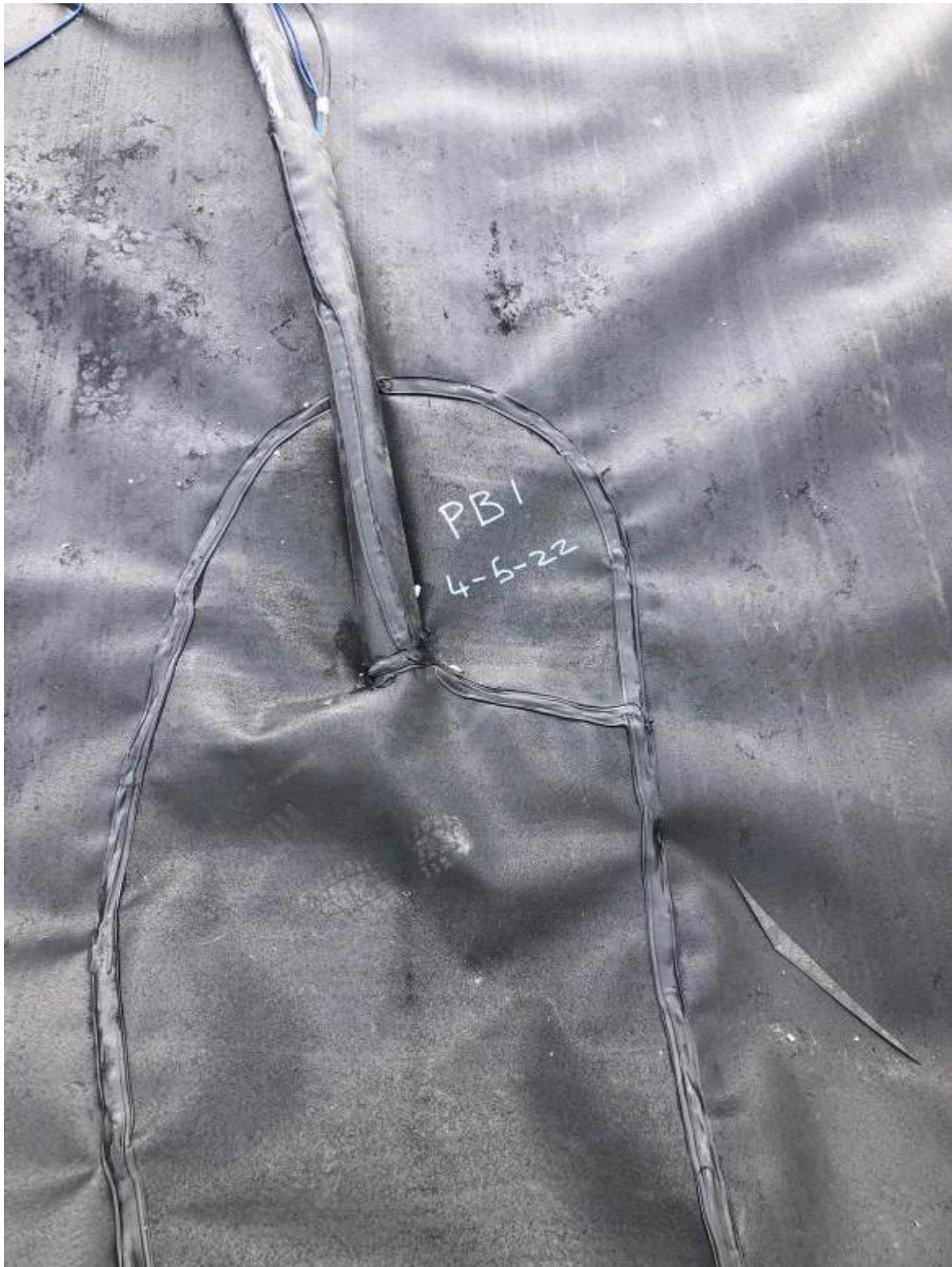
Pipe Boot Repair 1
