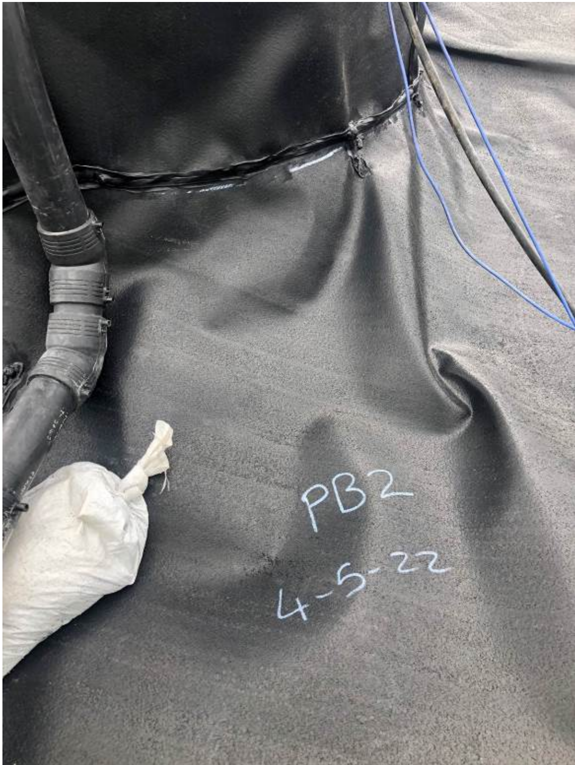
Pipe Boot Repair 2
