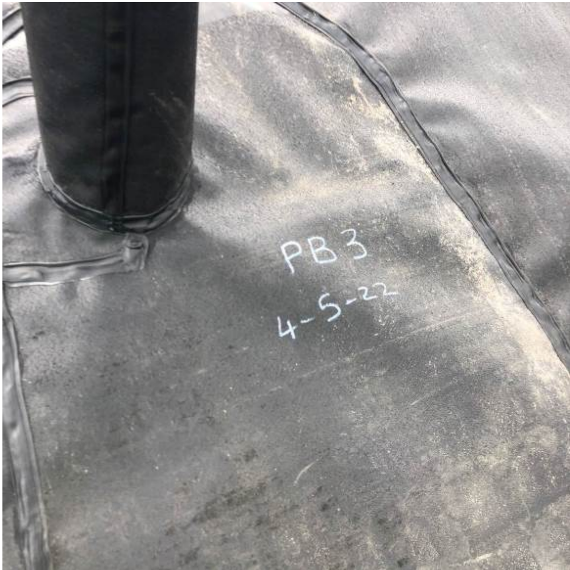
Pipe Boot Repair 3
