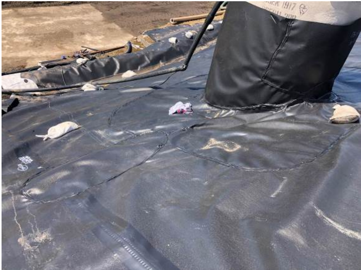
Pipe Boot Repair 12
