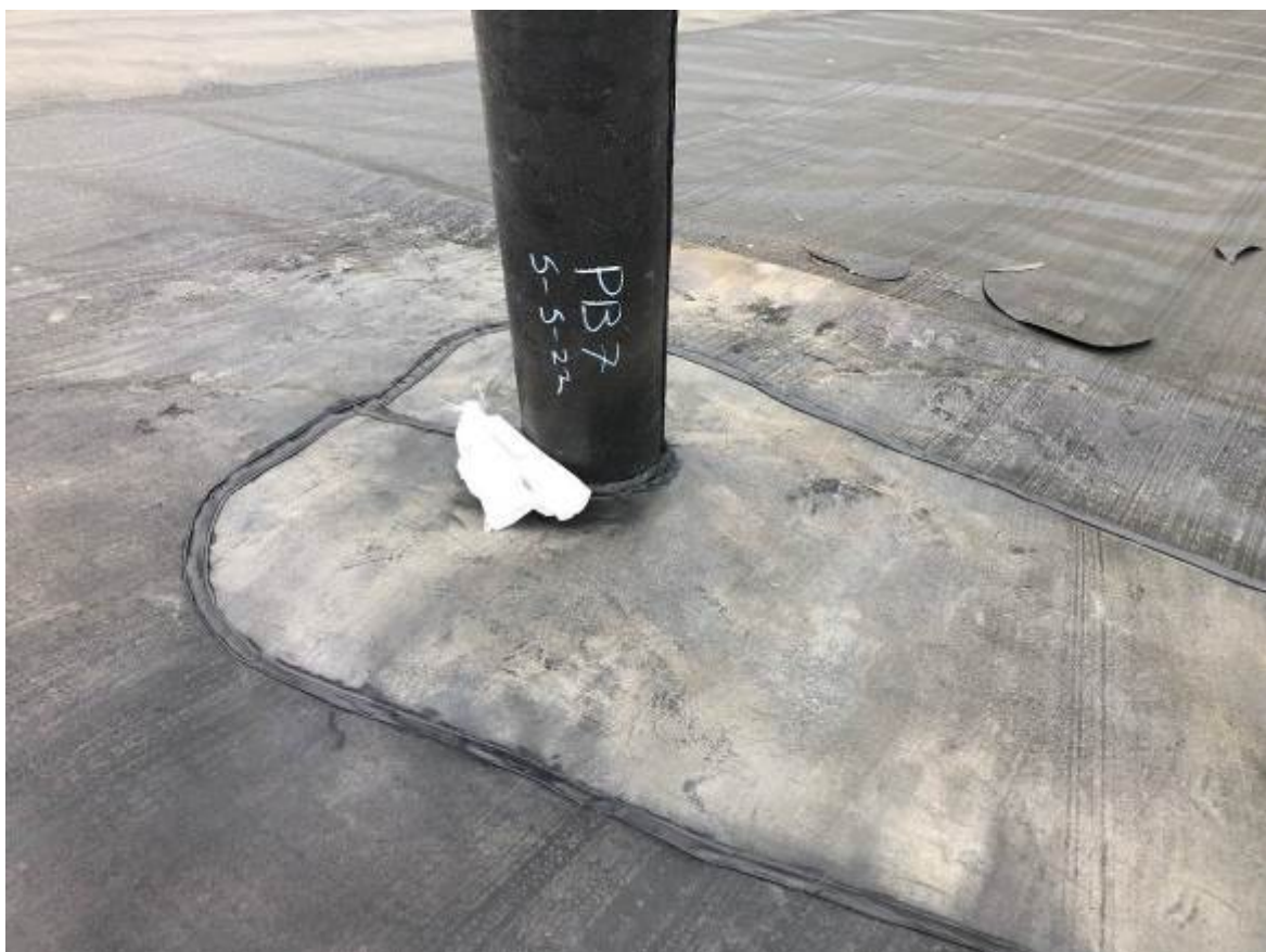
Pipe Boot Repair 7
