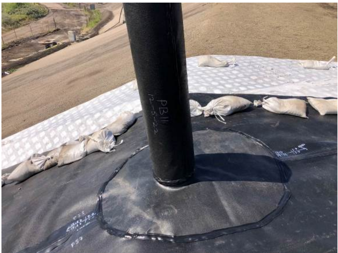
Pipe Boot Repair 11
