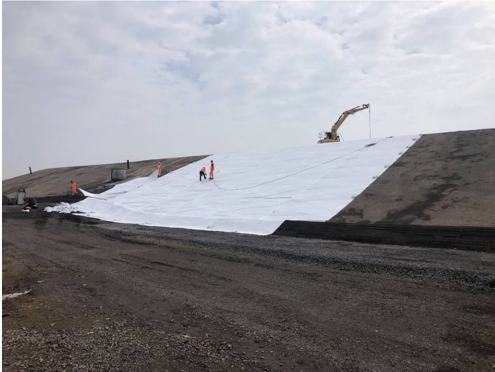
Placement of Gas Geocomposite on Eastern Flank
