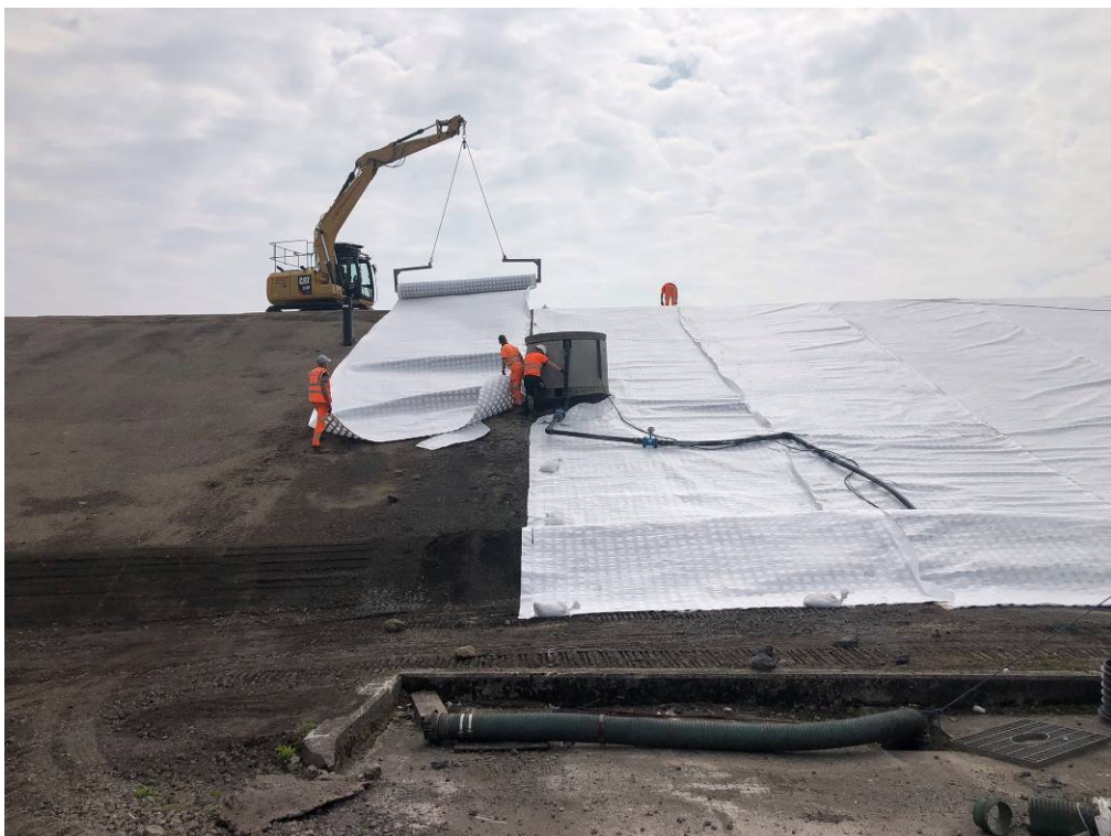
Placement of Gas Geocomposite around leachate extraction chamber
