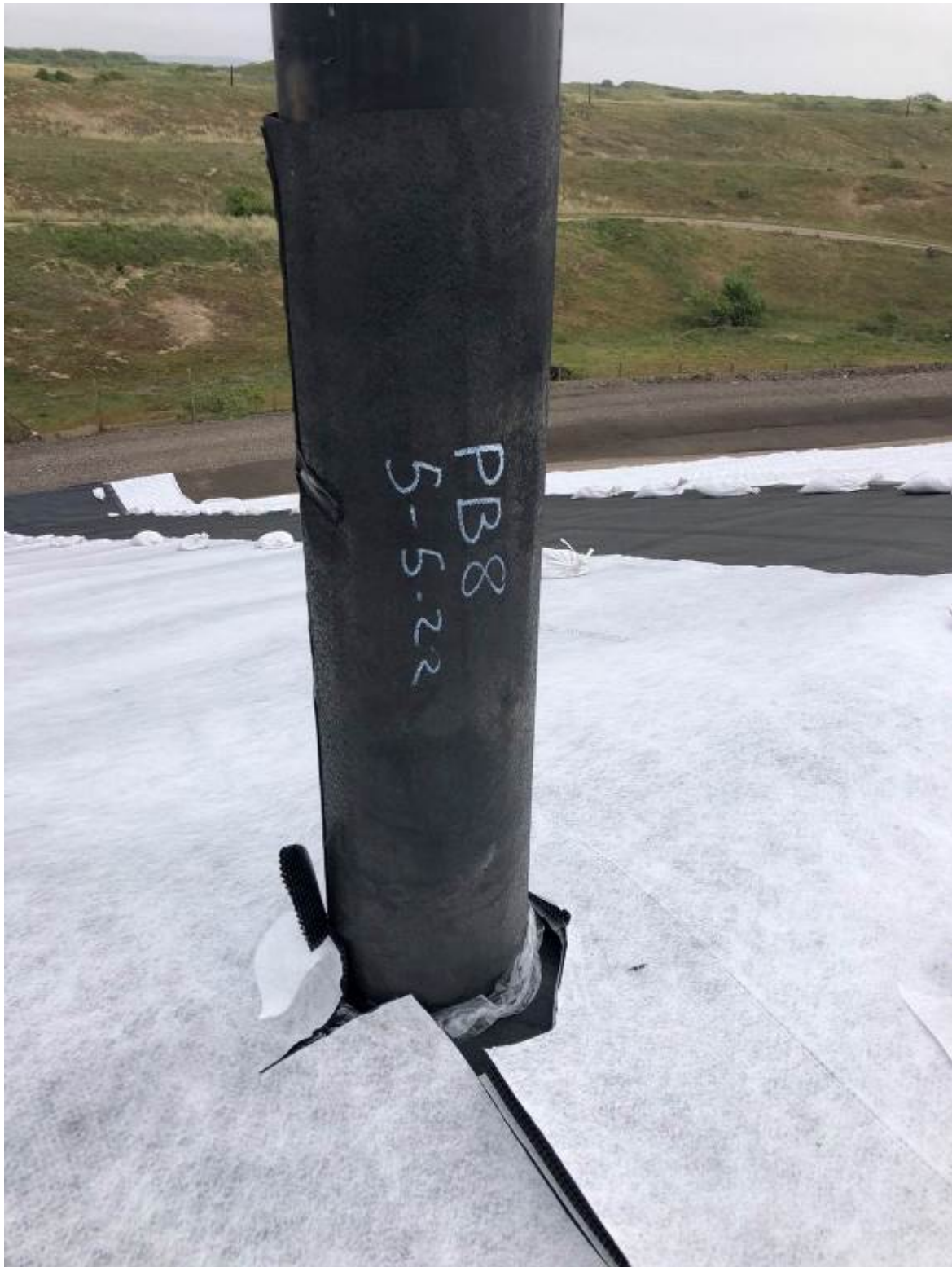
Pipe Boot Repair 8
