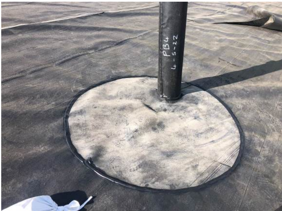
Pipe Boot Repair 5
