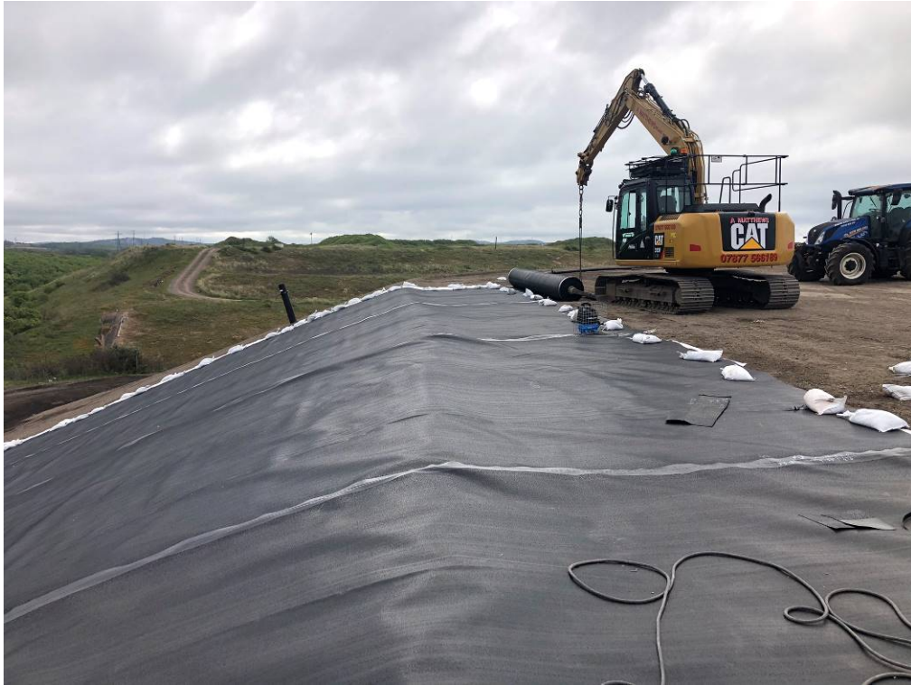
Vacuum Box Testing
