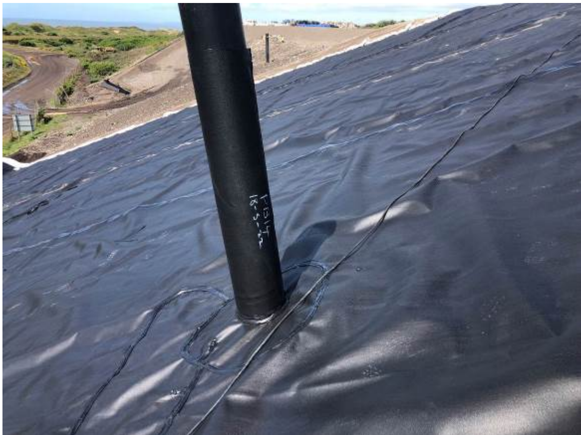
Pipe Boot Repair 14
