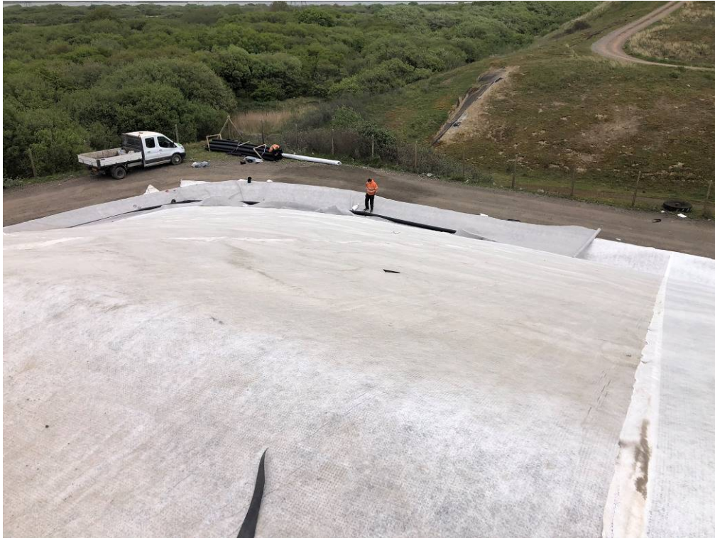
Surfacewater Geocomposite Placement
