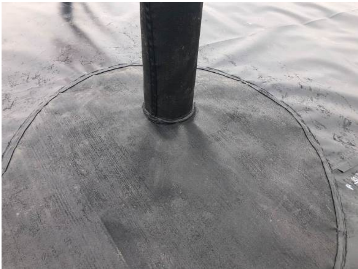
Pipe Boot Repair 13
