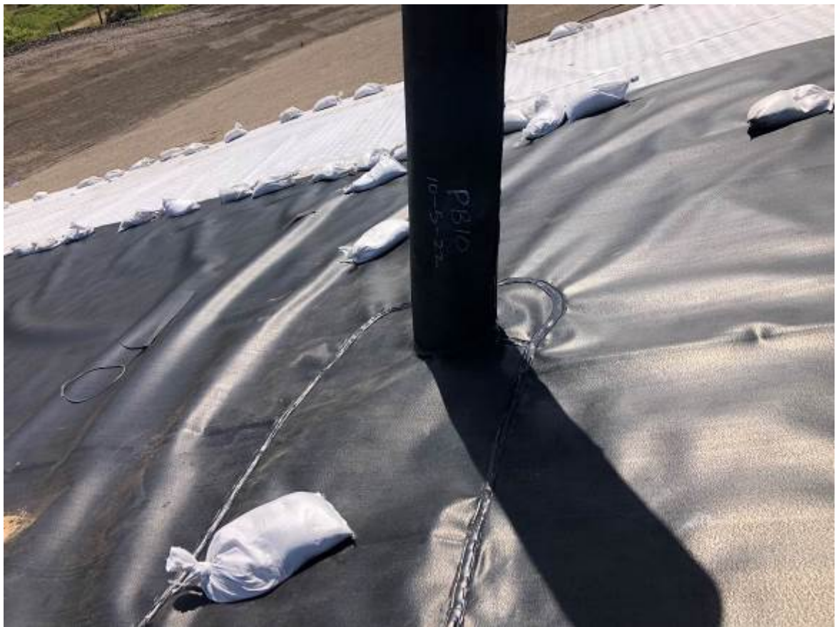
Pipe Boot Repair 10
