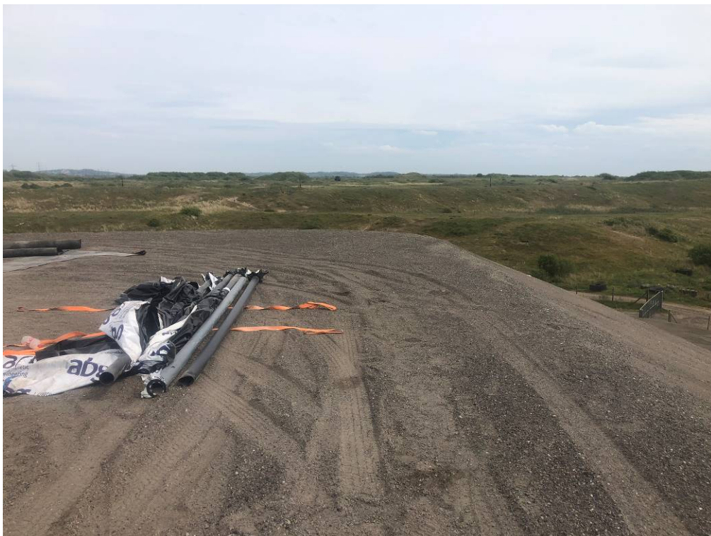
Placement of Dust Regulating Layer
