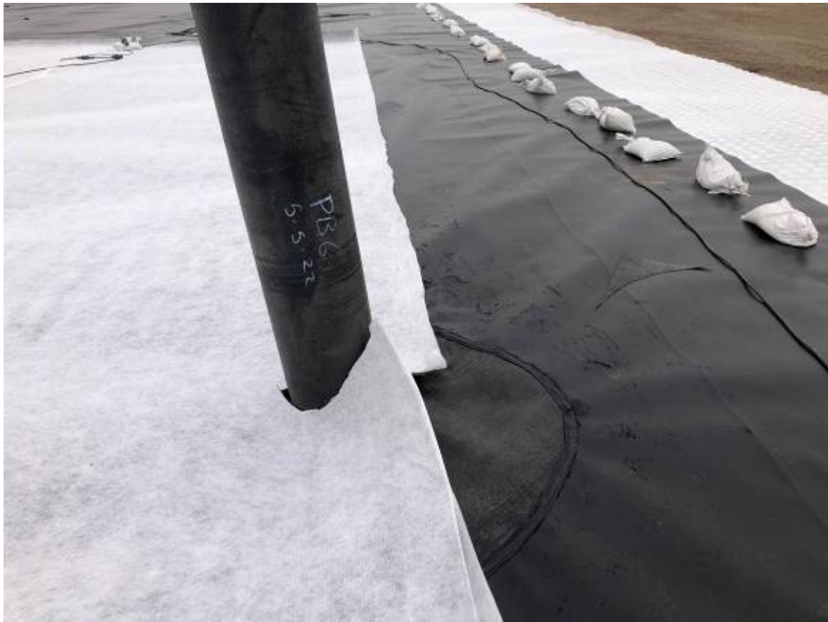
Pipe Boot Repair 6
