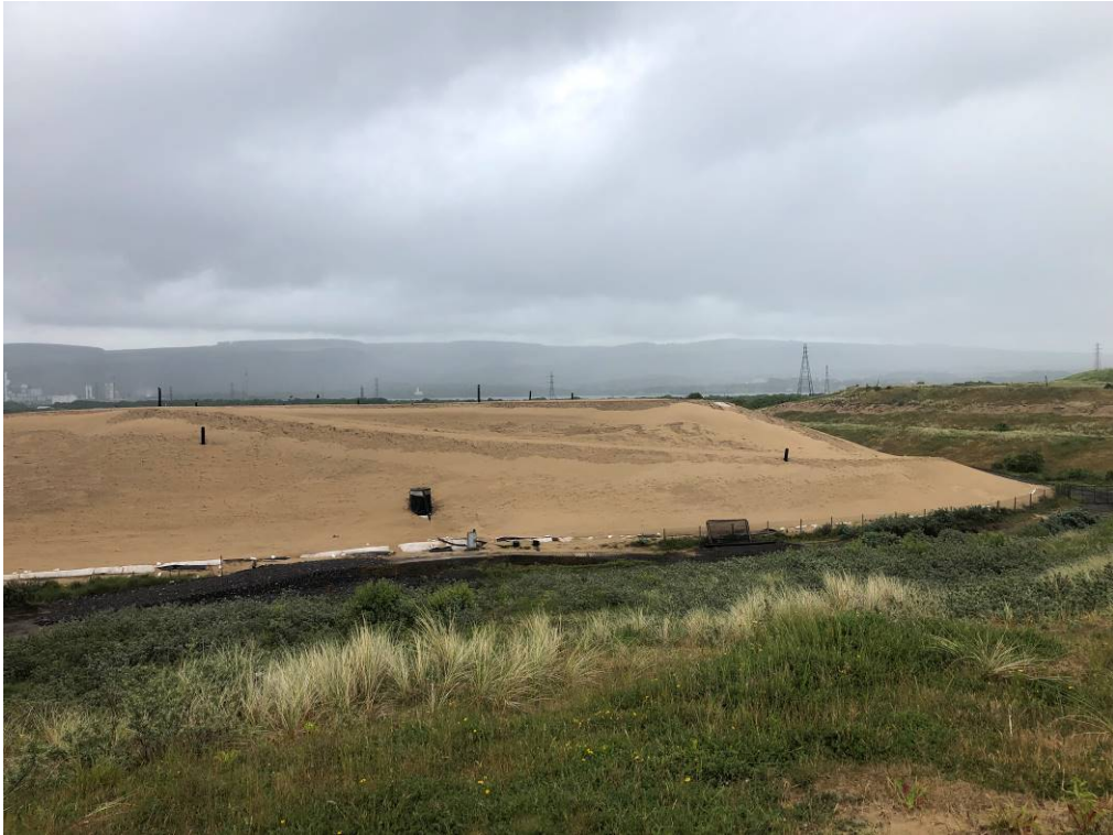
Biocell covered in restoration soil (sand)
