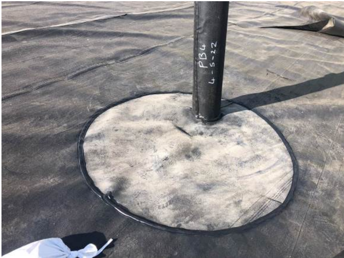
Pipe Boot Repair 4
