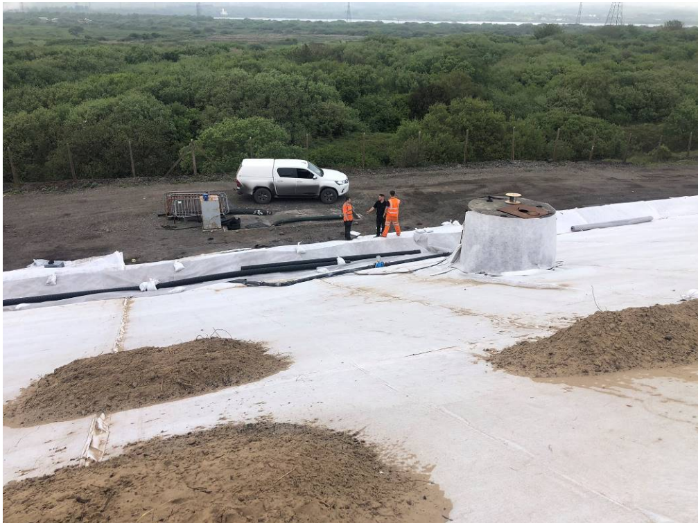
Surfacewater Geocomposite secured by restoration soils
