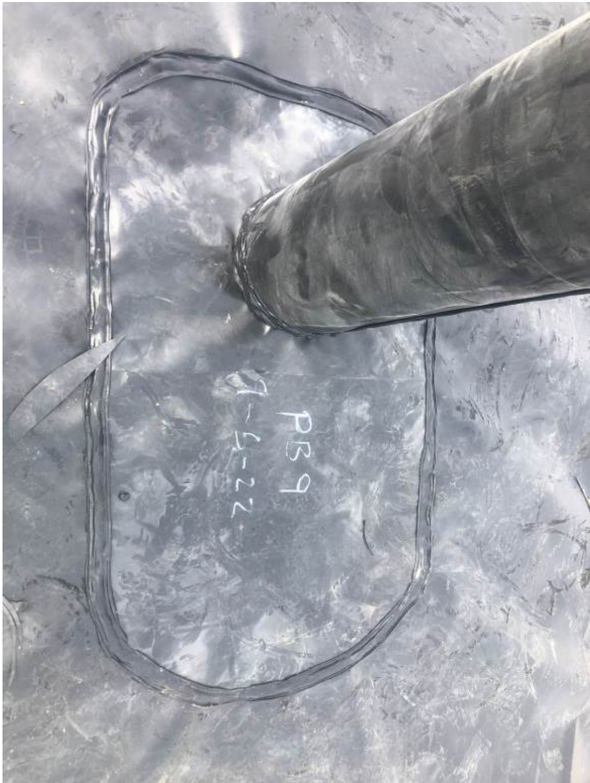
Pipe Boot Repair 9
