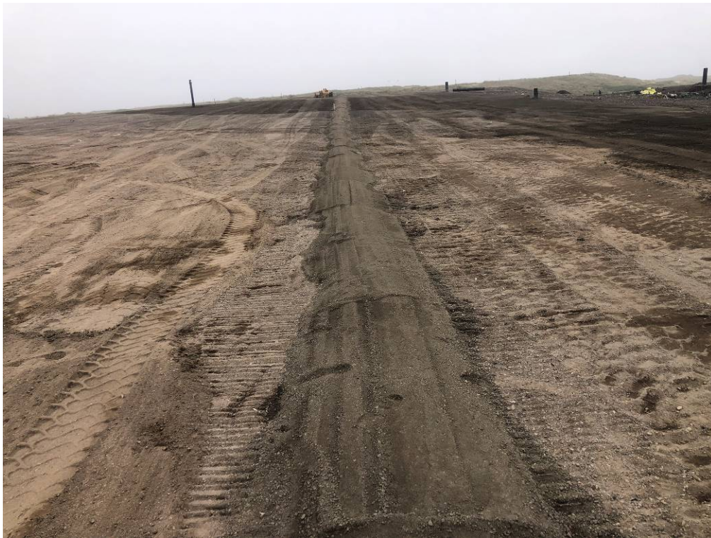
Placement of regulating layer
