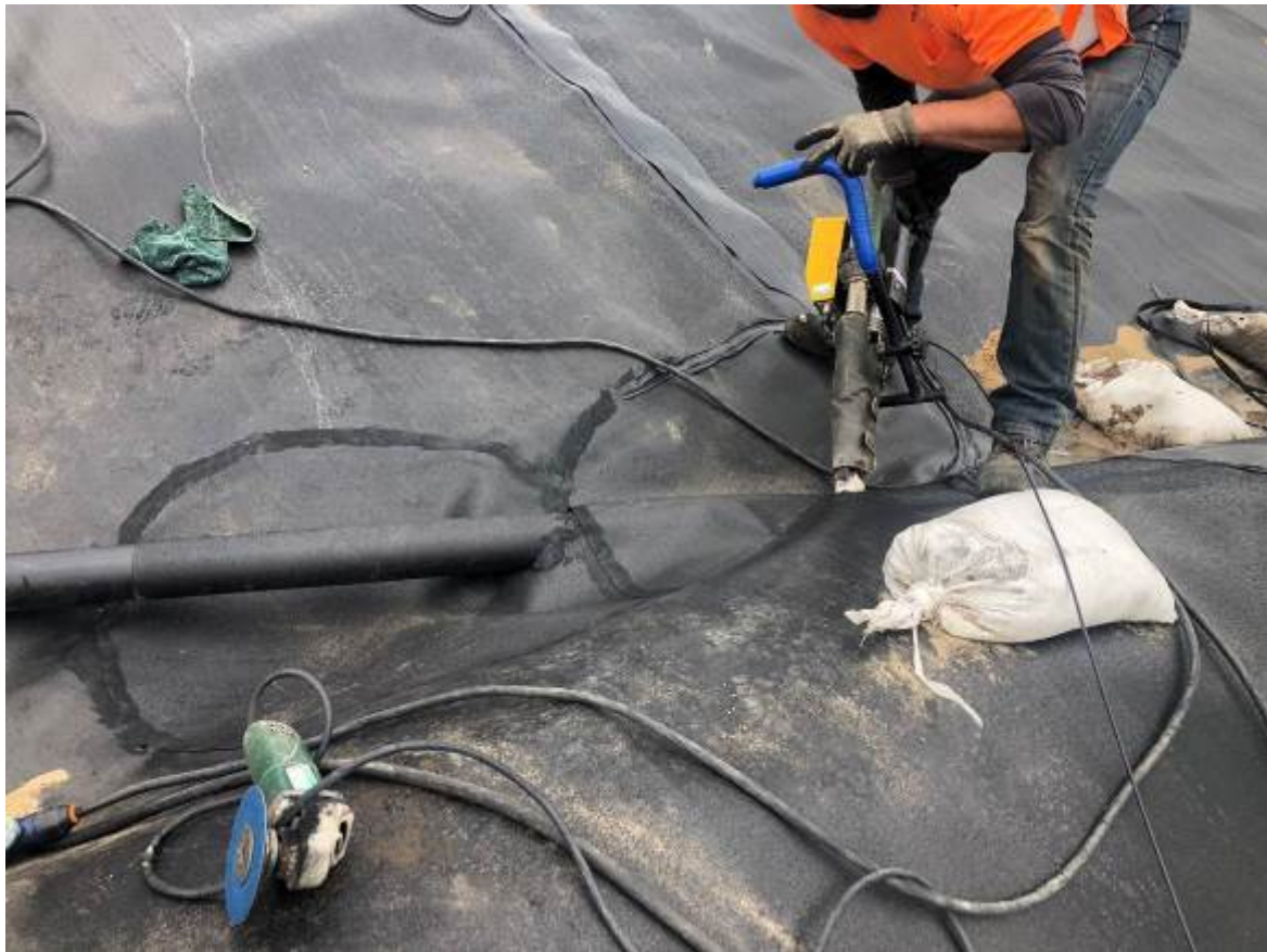
Pipe Boot Repair 16
