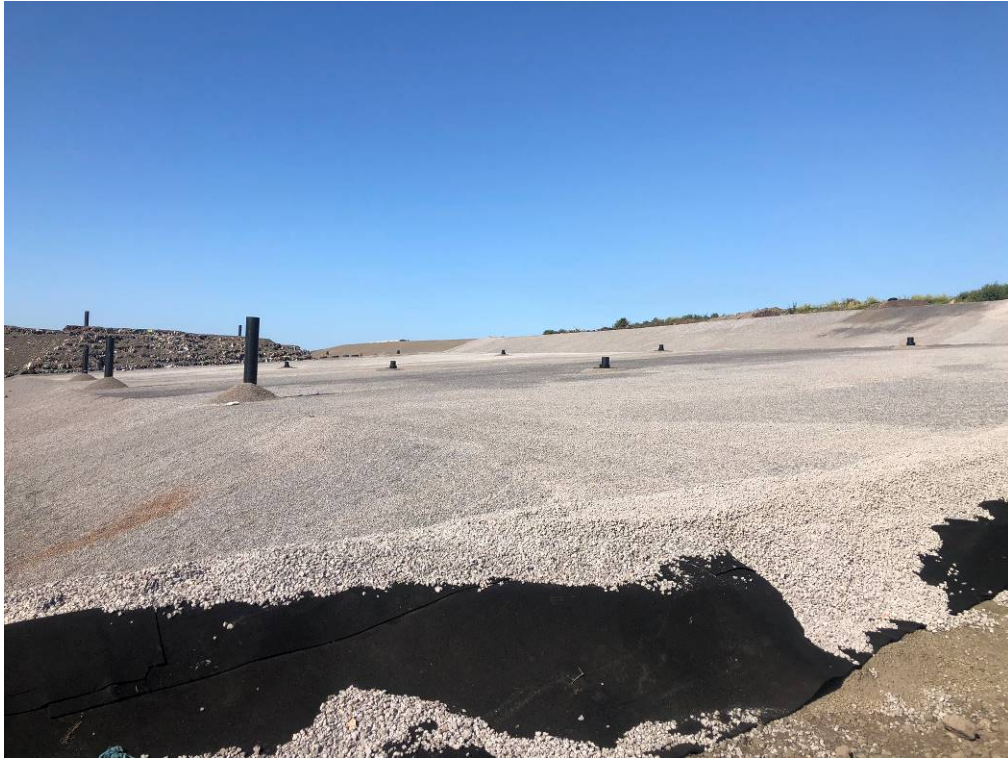
Completed drainage layer with base gas wells in-situ
