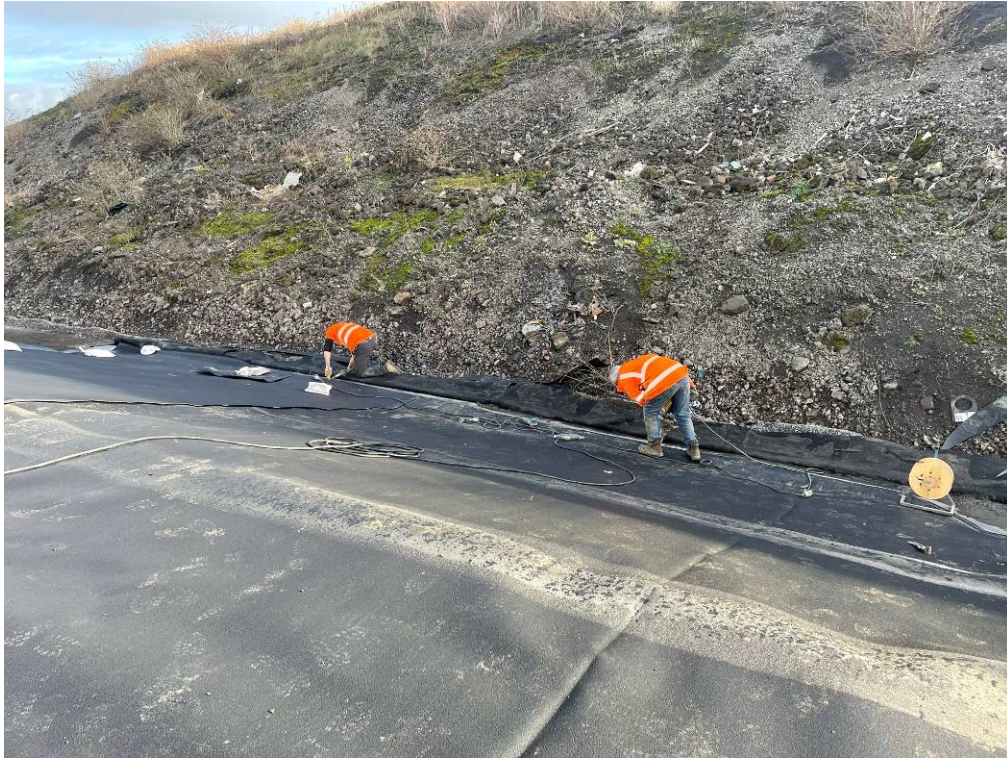
Extrusion welding at toe of slope
