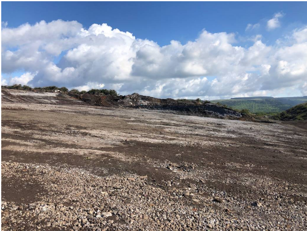
Excavation of Formation
