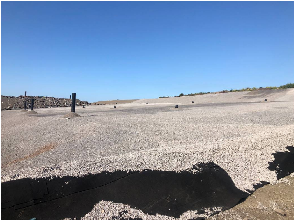
Gas Well Installation in Bio-cell Extension B
