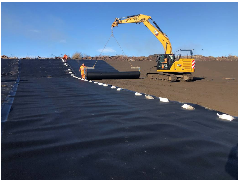
Placement of HDPE
