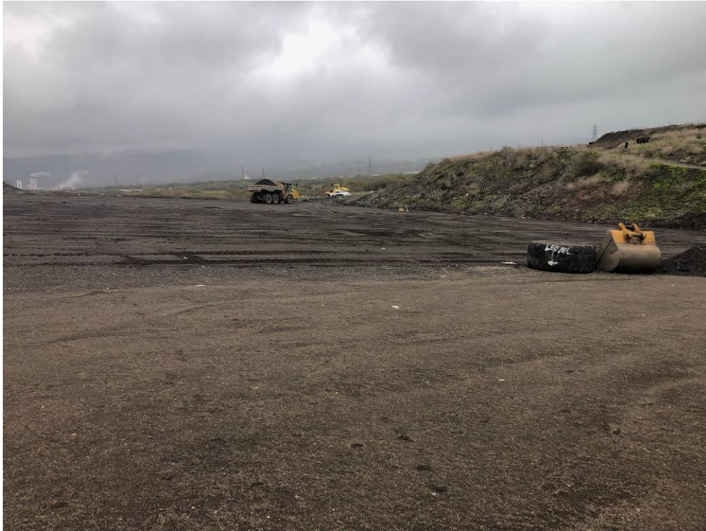
Placement of Dust Regulating Layer
