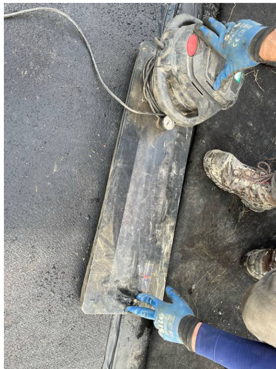
Vacuum Box Testing
