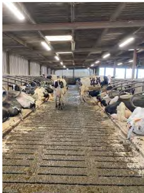
Figure 7: cubicles with rubber mattresses topped with sawdust. This shed has slatted floors in the passageways to remove slurry.
