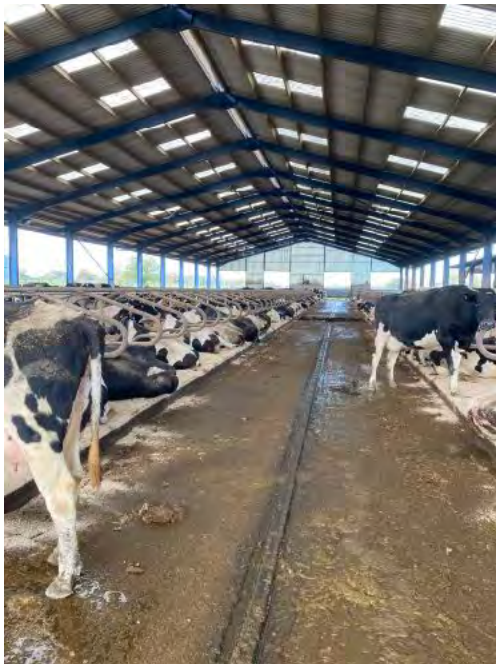
Figure 6: cubicles with rubber mattresses topped with sawdust. This shed has solid floors and automatic scrapers in the passageways to remove slurry.
