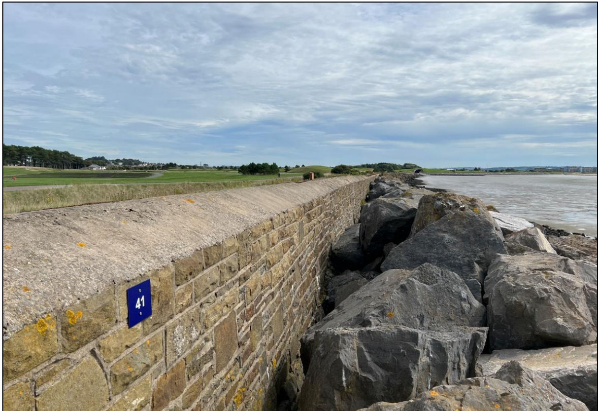
Figure 9: Seawall defence protected by significant rock armour embankment.
