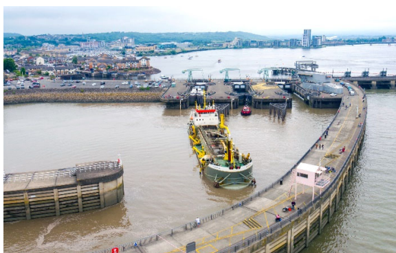
Figure 1 - Sospan Dau completing works within the Outer Harbour
