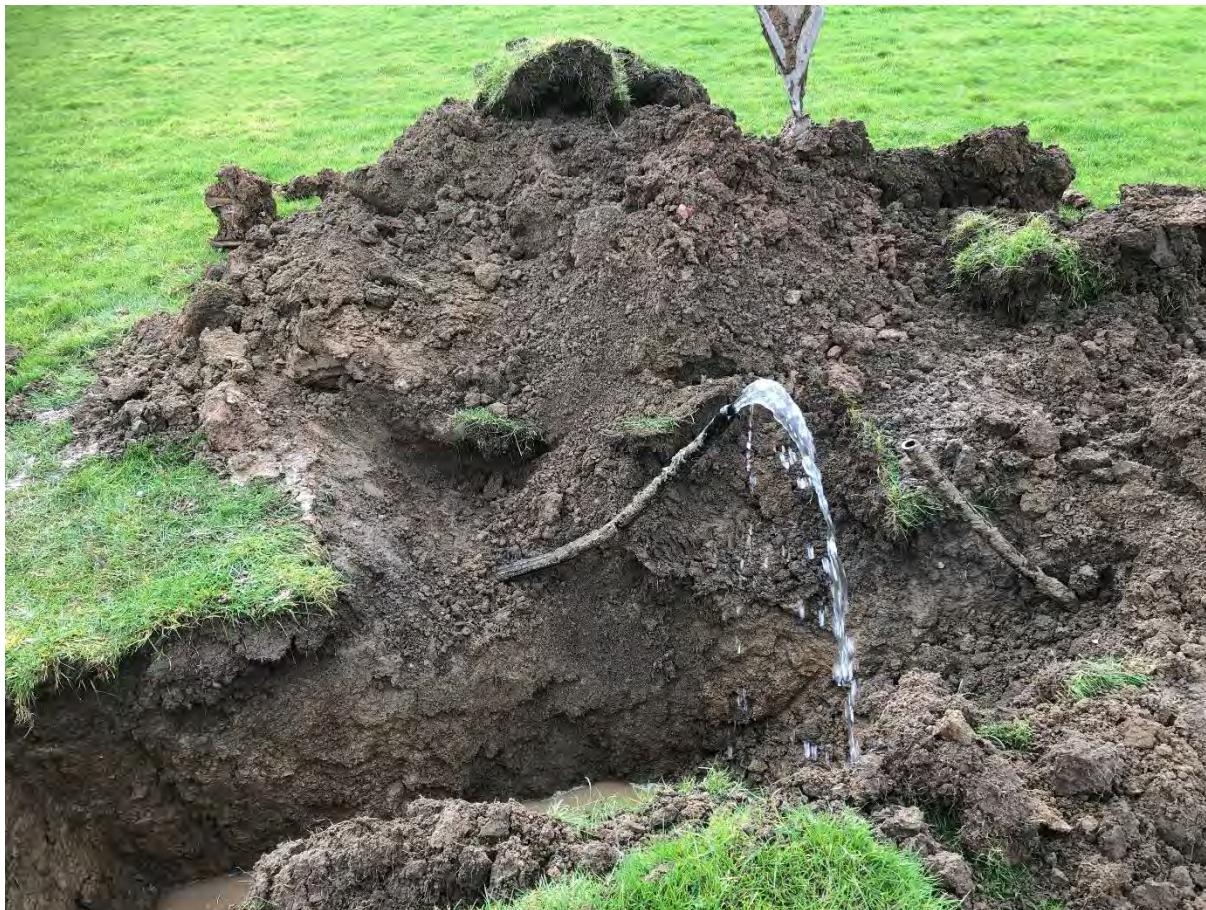
TP109 Soil arisings. Buried water line set at 0.35mbgl. Pipe fully repaired before reburying and reinstatement works Trial pit base set at 1mbgl on stiff clay (HSV at 1mbgl = 110 Cu(kN/m 2 ))
