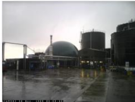
P17 AD plant
