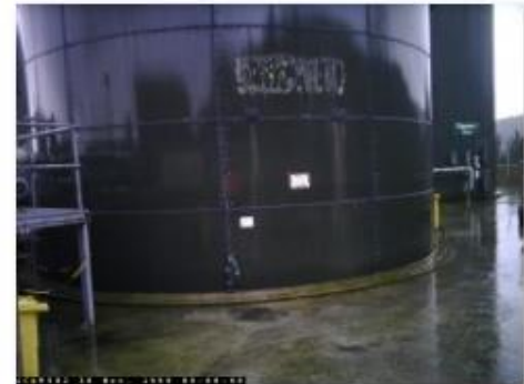
P18 RWB tank
