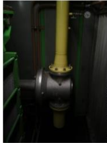
P56 CHP unit gas incomer
