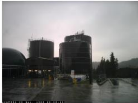
P16 AD plant
