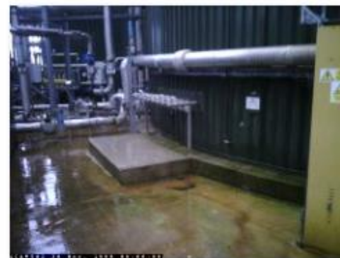
P27 gas mixing system removed from a process vessel
