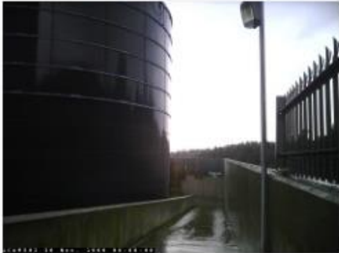
P40 digestate storage tank
