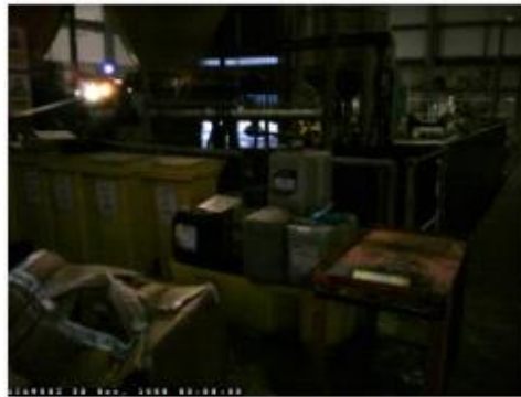
P5 chemicals and lubricants in reception hall
