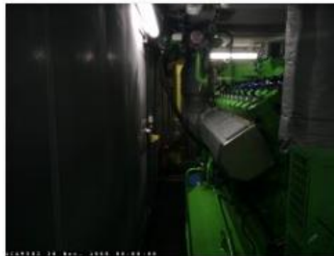
P59 CHP unit enclosure and gas alarm and e-stop
