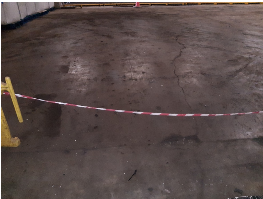
Photo 3 – visible cracking in the area where the reception bays were located.
