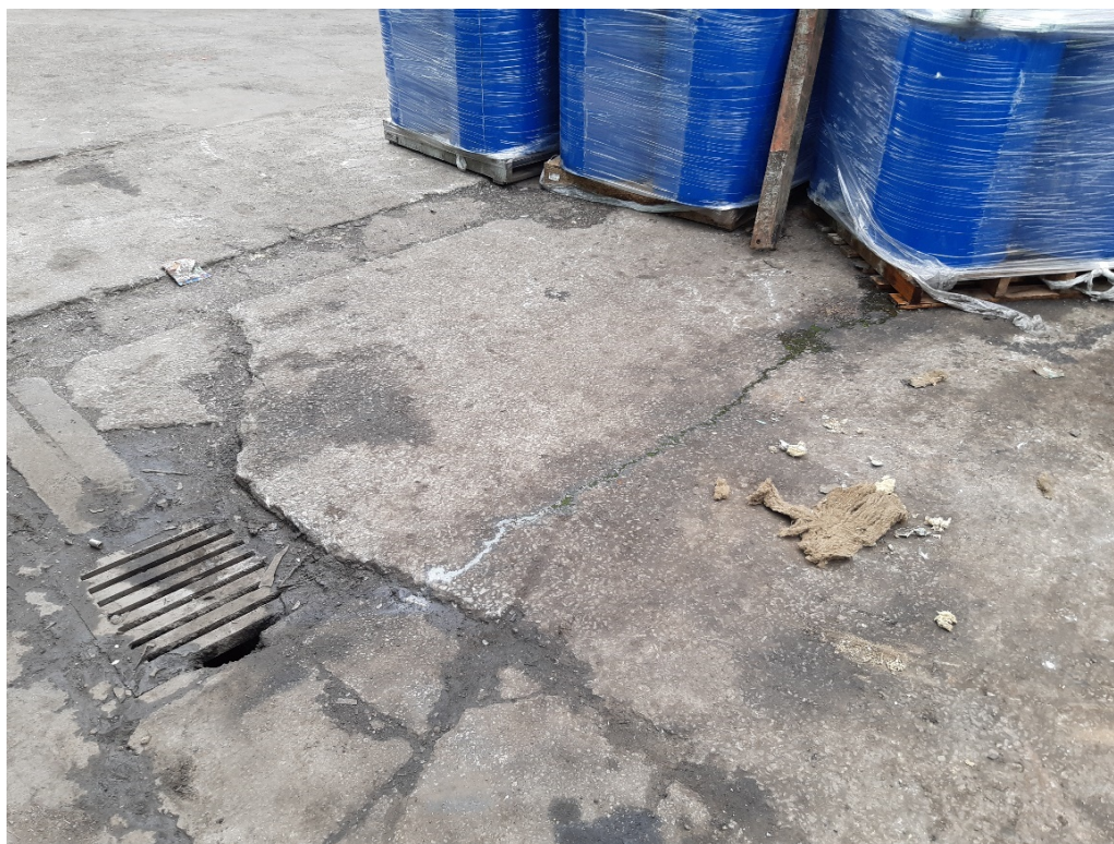
Photo 1 – unknown liquid migrating towards surface water drains within yard area outside main building.
