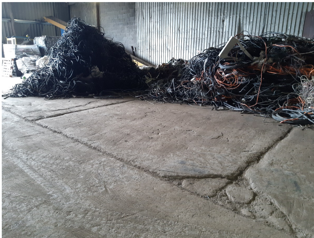
Photo 4 – deterioration of concrete surface within the cable storage area.
