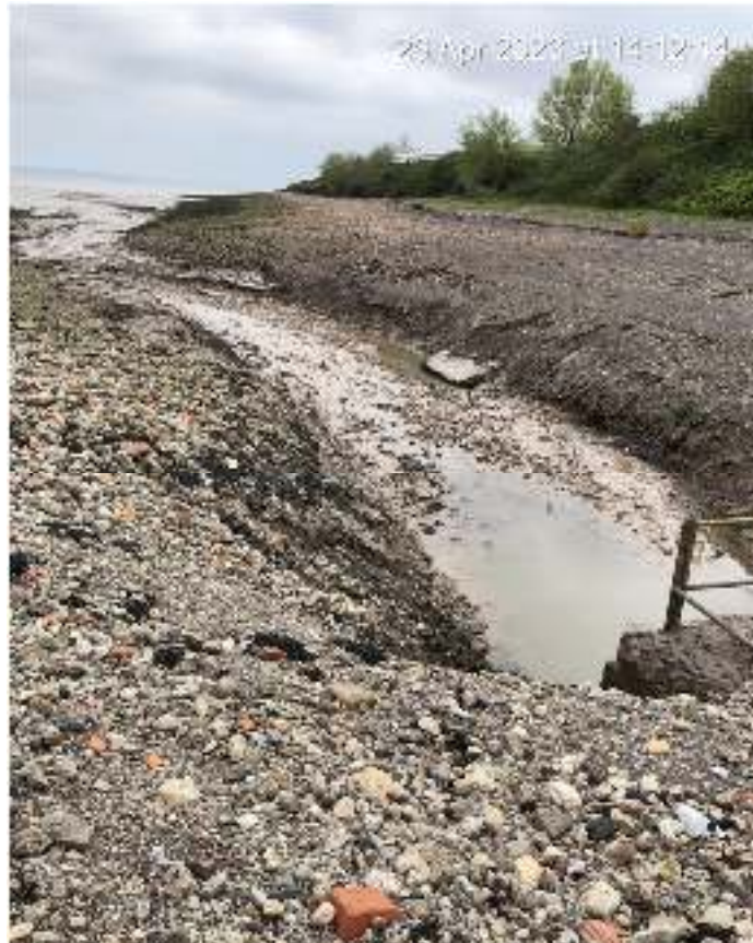
Figure 5 – outfall location looking out to estuary.
