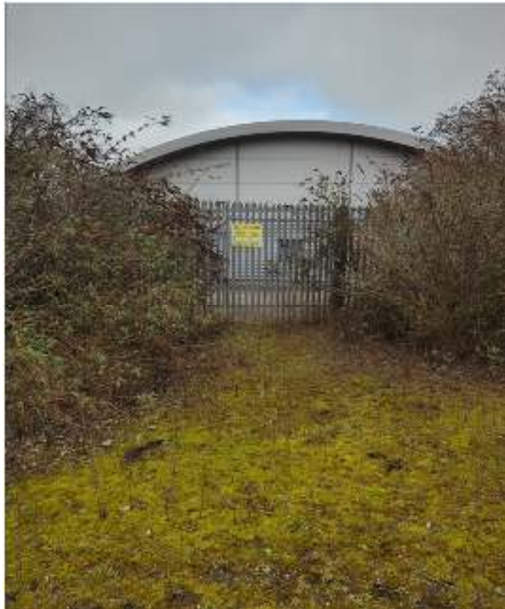
Figure 3 – access gate from WWTW.
