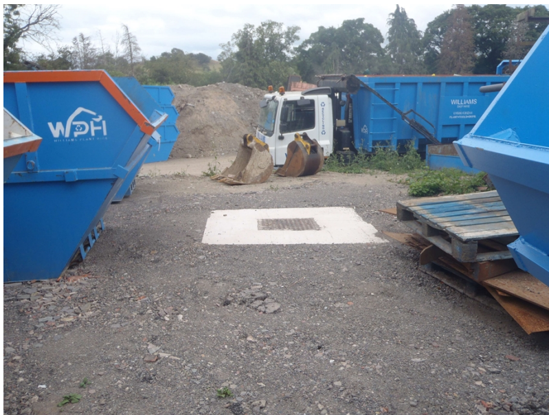
Inspection chamber for tank
