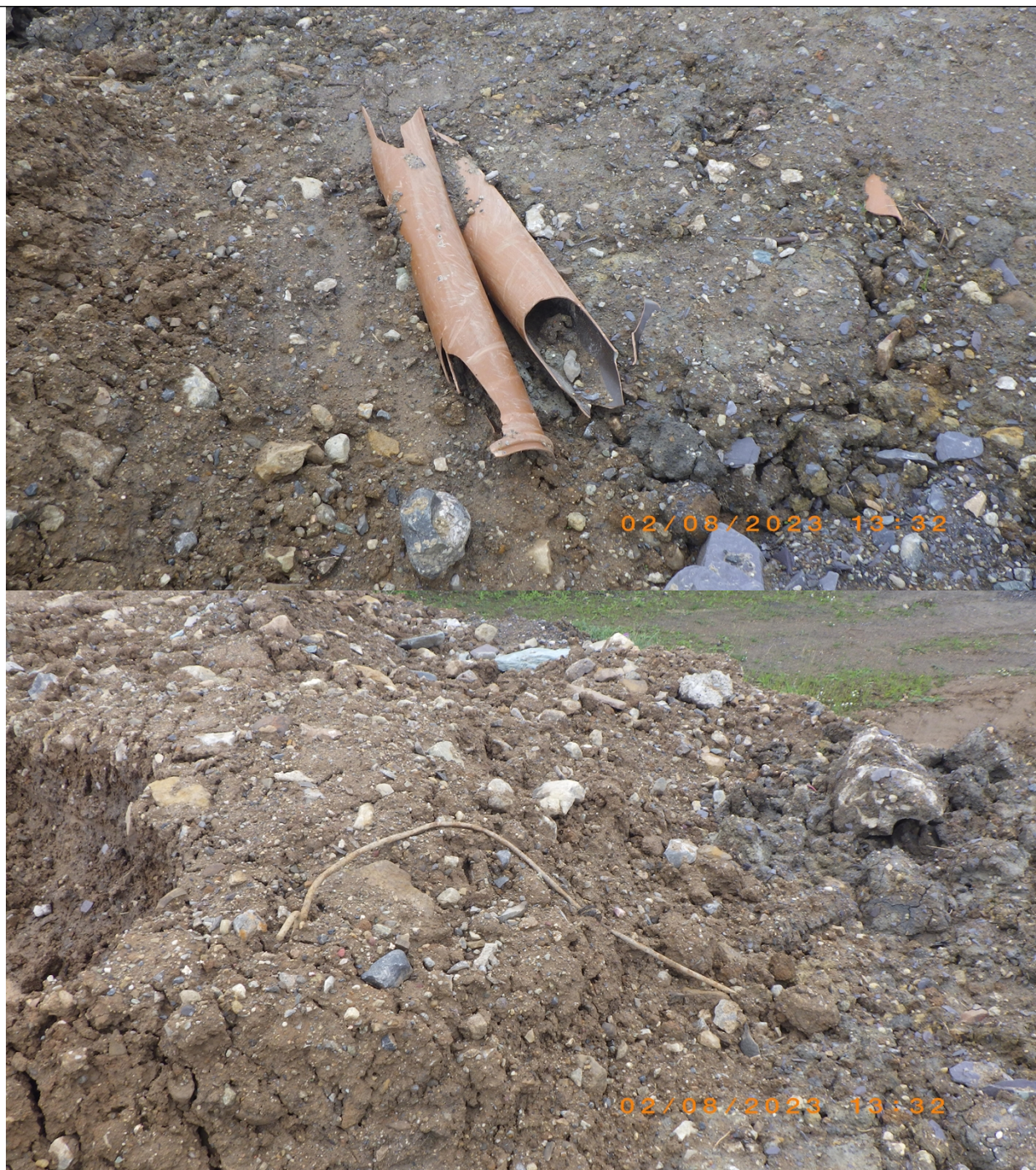
Photos showing deposited waste containing plastics and metals, within the current working cell.
