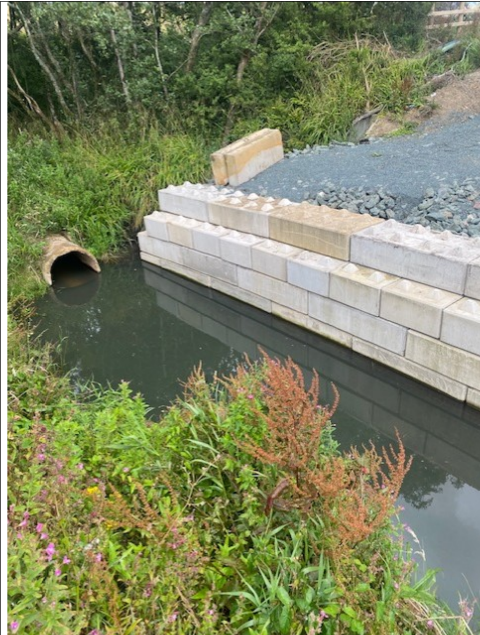
Figure 2 - Culvert Completed Works Upstream
