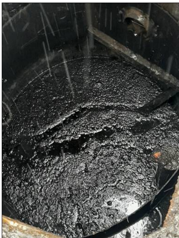
Image 11 - showing the contents of the operator's interceptor holding large volumes of oils and fuels - taken by Officer Chris BURGE at 12:01 on 9 September 2021
