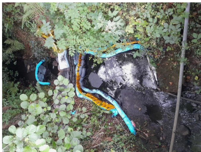
Image 10 - showing containment measures capturing oils and fuels in the unnamed tributary of the Nant Cylla downstream from the site - taken by Officer Alex BOWDER at 10:07 on 3 September 2021
