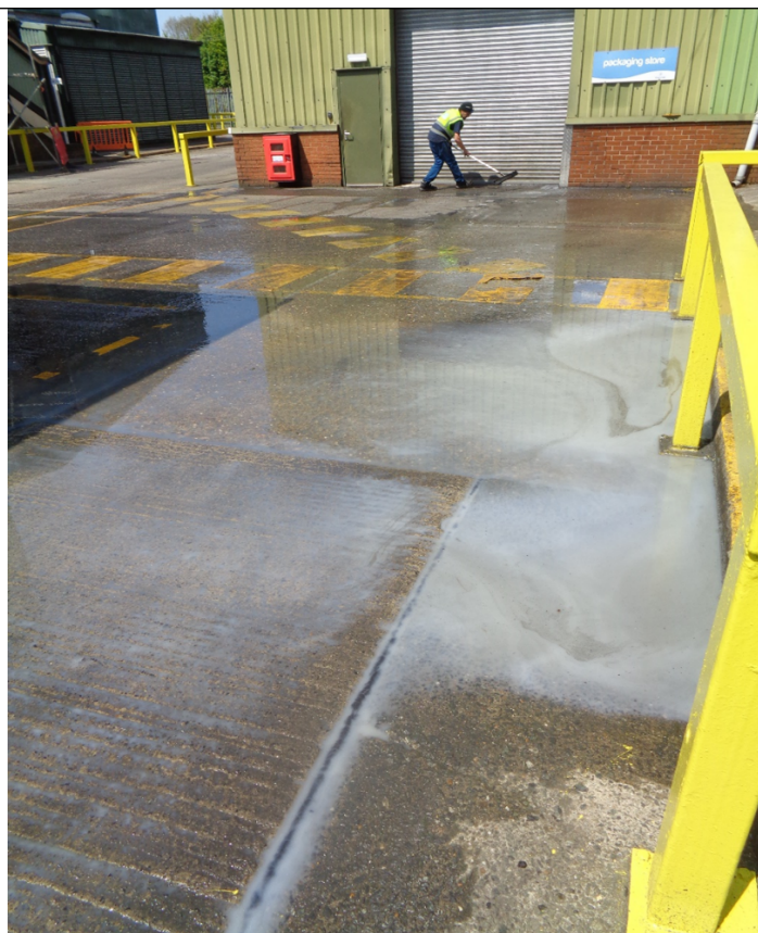
Fig 2 above. Taken on 22 nd May 2023 by visiting EHO PCC food safety team. Shows milky effluent pooling in the First Milk yards. This acts as a possible source of high COD/BOD pollution if left to overflow off site.
