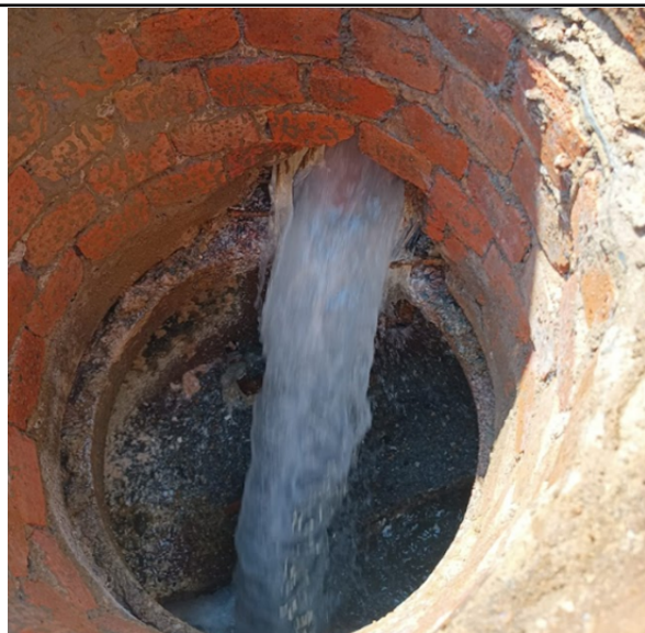
Fig 3 Dwr Cymru gravity fed drain SM94149502 taken by Dwr Cymru staff shows milky effluent entering their drain on 7th June through an unpermitted emission point inside First Milks site boundary.
