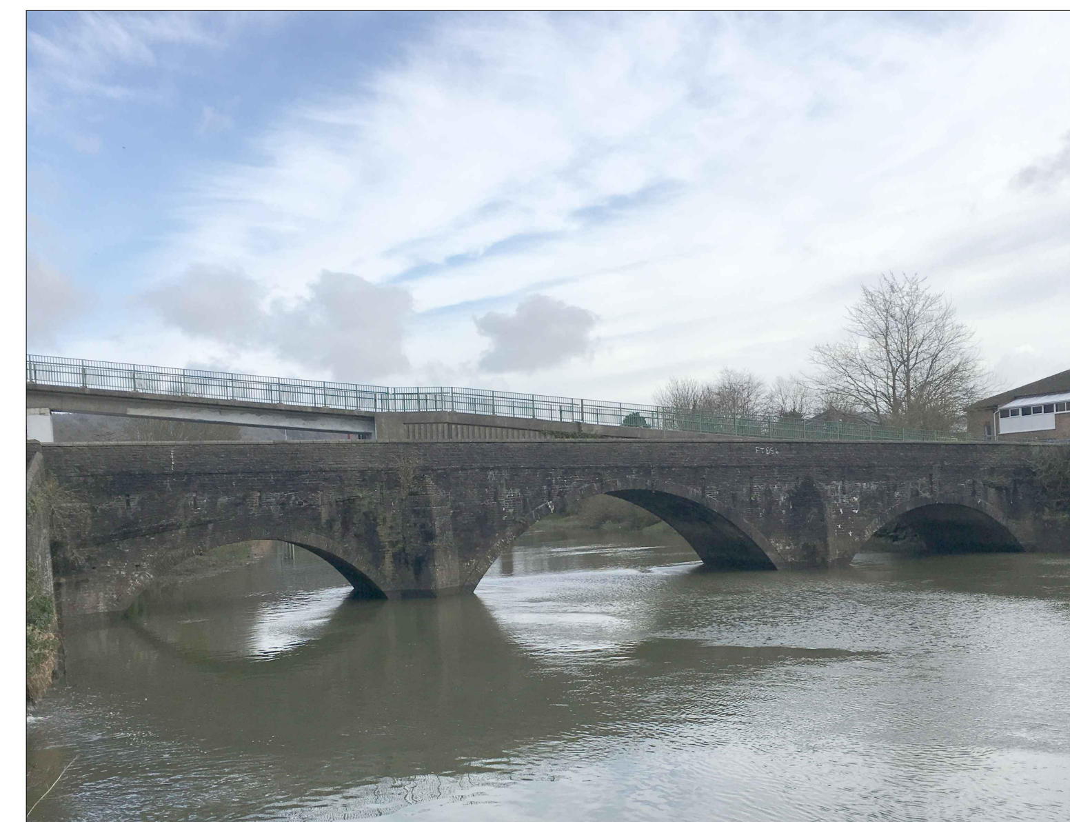
STRUCTURE PHOTOGRAPHS NTS
