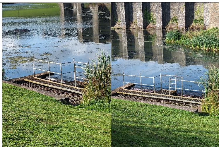
Figure 2 and 3. Surrounding area of water outlet.
