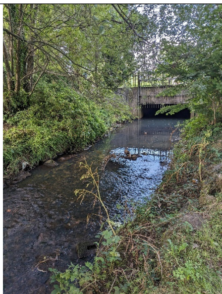
Figure 5. The culvert where the outlet discharges into Porset Brook.
