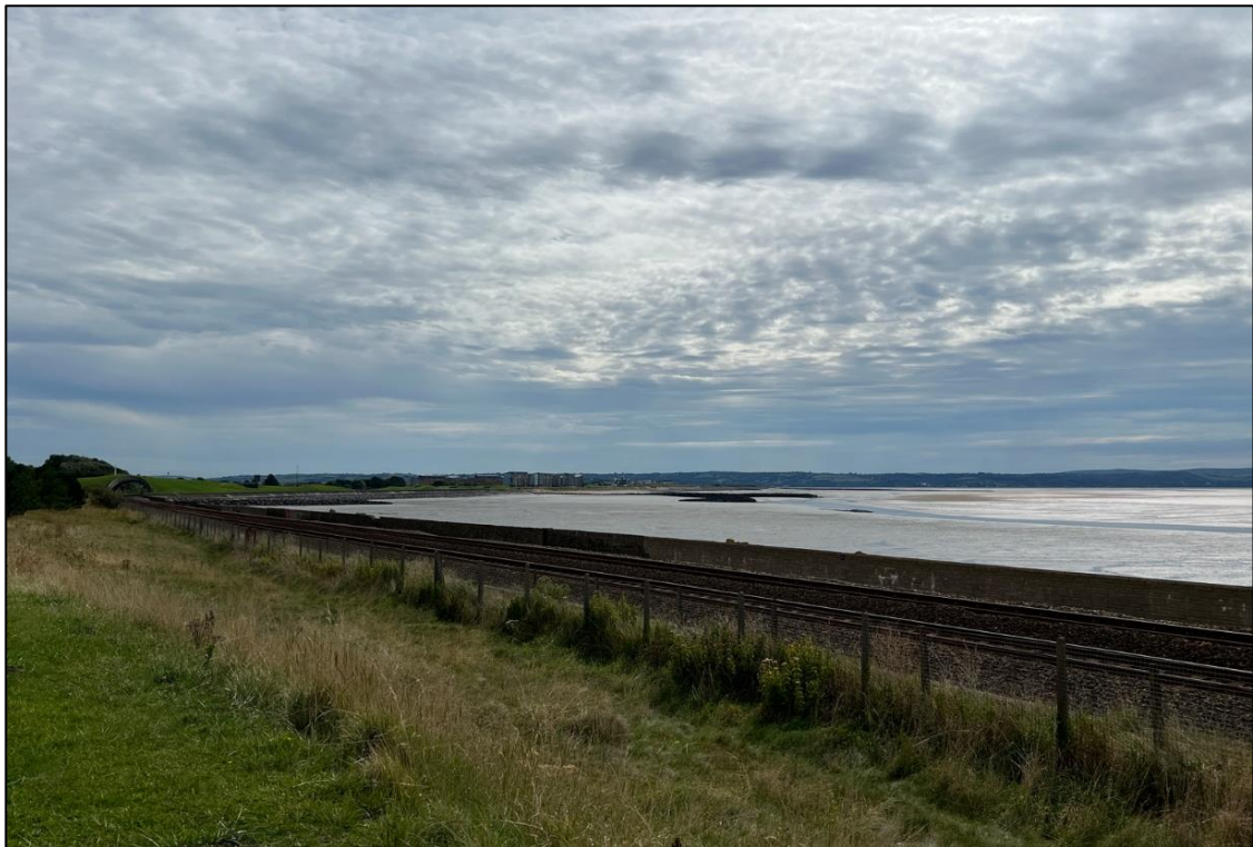
Figure 8: Rear of sea wall behind network rail boundary.
