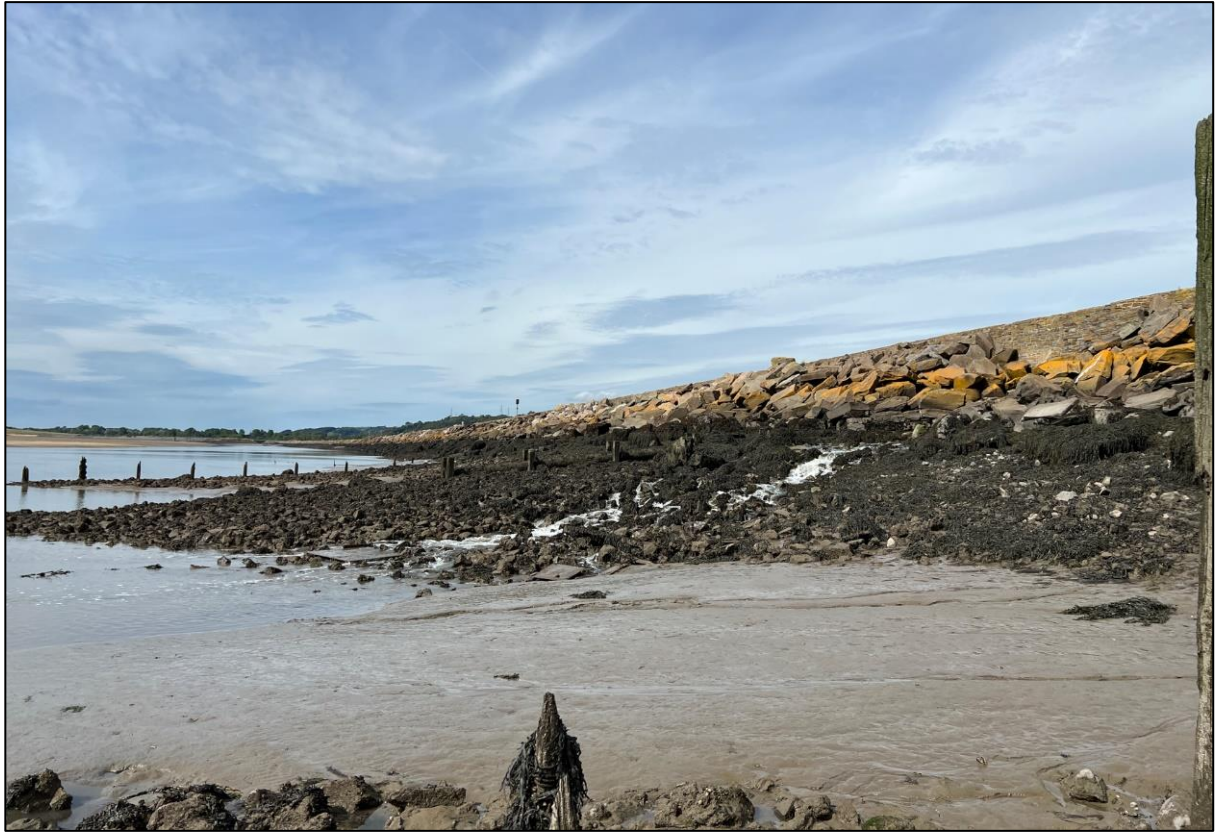
Figure 11: Outfall situated between rock armour and defence wall.
