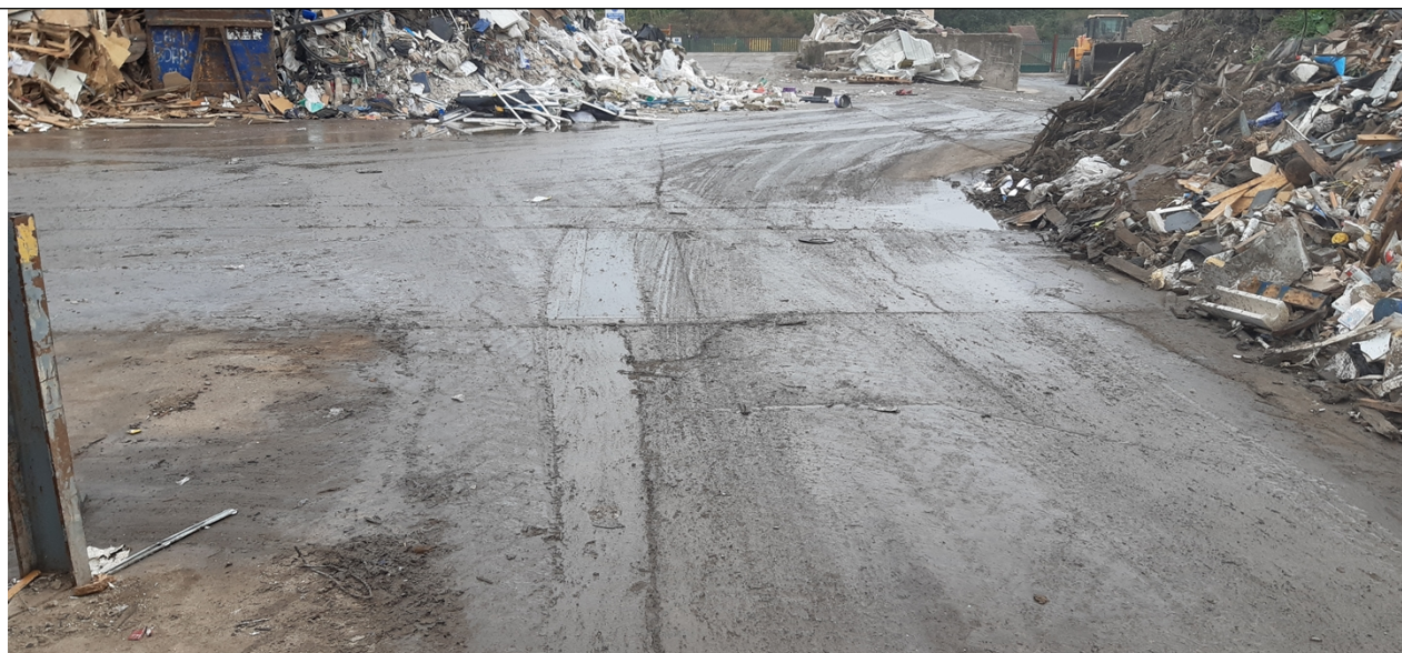
Photo 3 - Improved areas of flooring infrastructure
