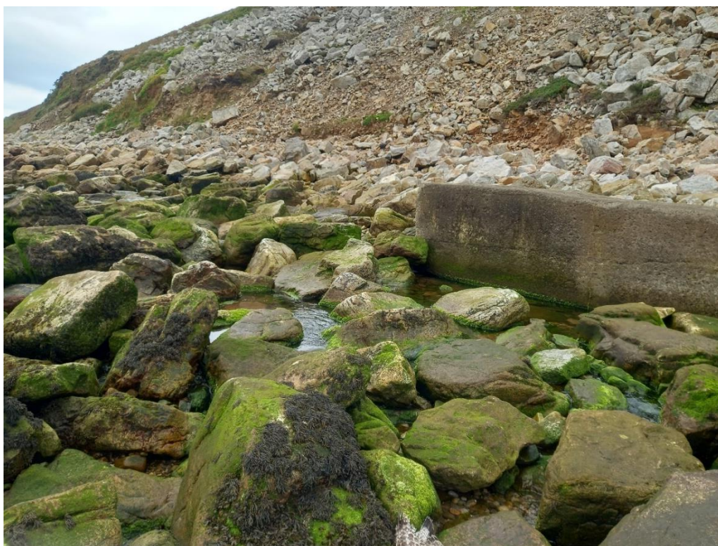
Rocky substrate to be levelled off and relocated from in front of the outfall.
