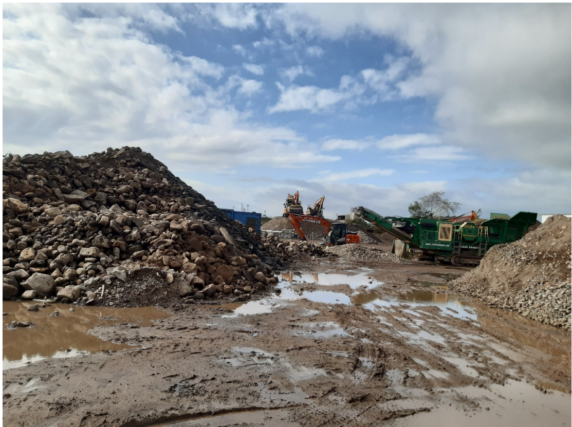
Photo 2 – Another photo showing area used for processing with mobile crusher in background
