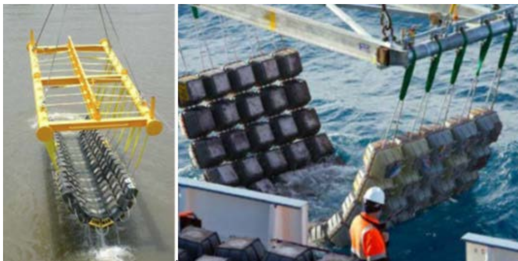
Figure 2-2 Figure 2-2 Concrete mattress deployment (courtesy of FoundOcean)
