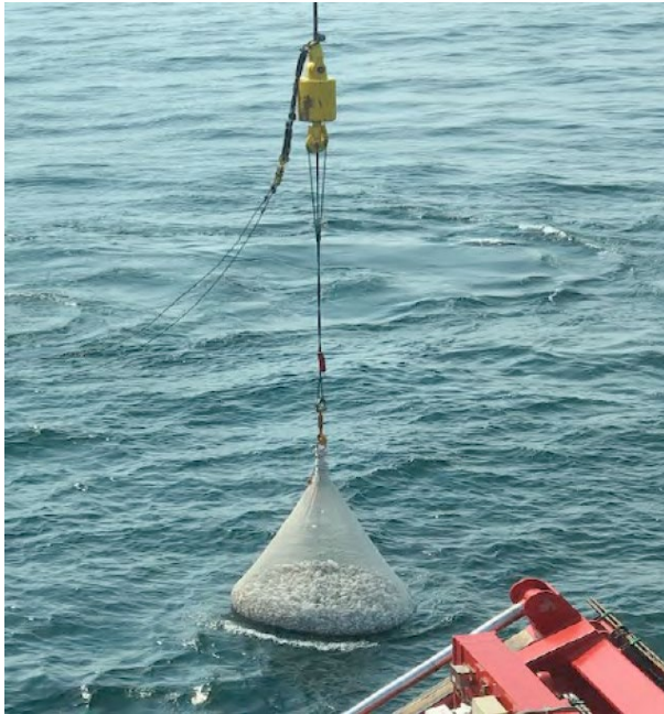
Figure 2-3 Figure 2-3 Rock bag deployment (NKT)
