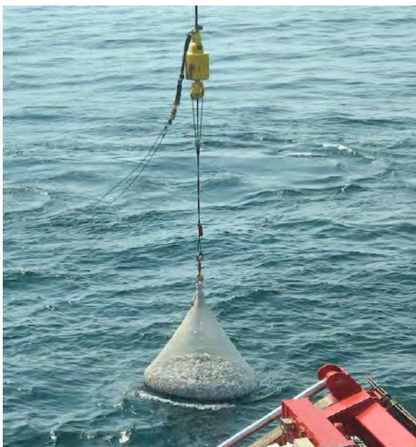
Figure 2-3 Figure 2-3 Rock bag deployment (NKT)
