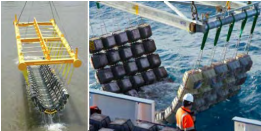
Figure 2-2 Figure 2-2 Concrete mattress deployment (courtesy of FoundOcean)
