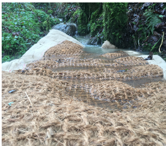
Each SiltMat can capture 40kg of sediment
