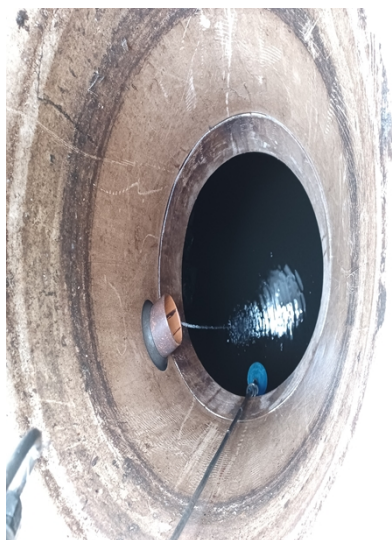
Photo 3 (Inside of chamber)
