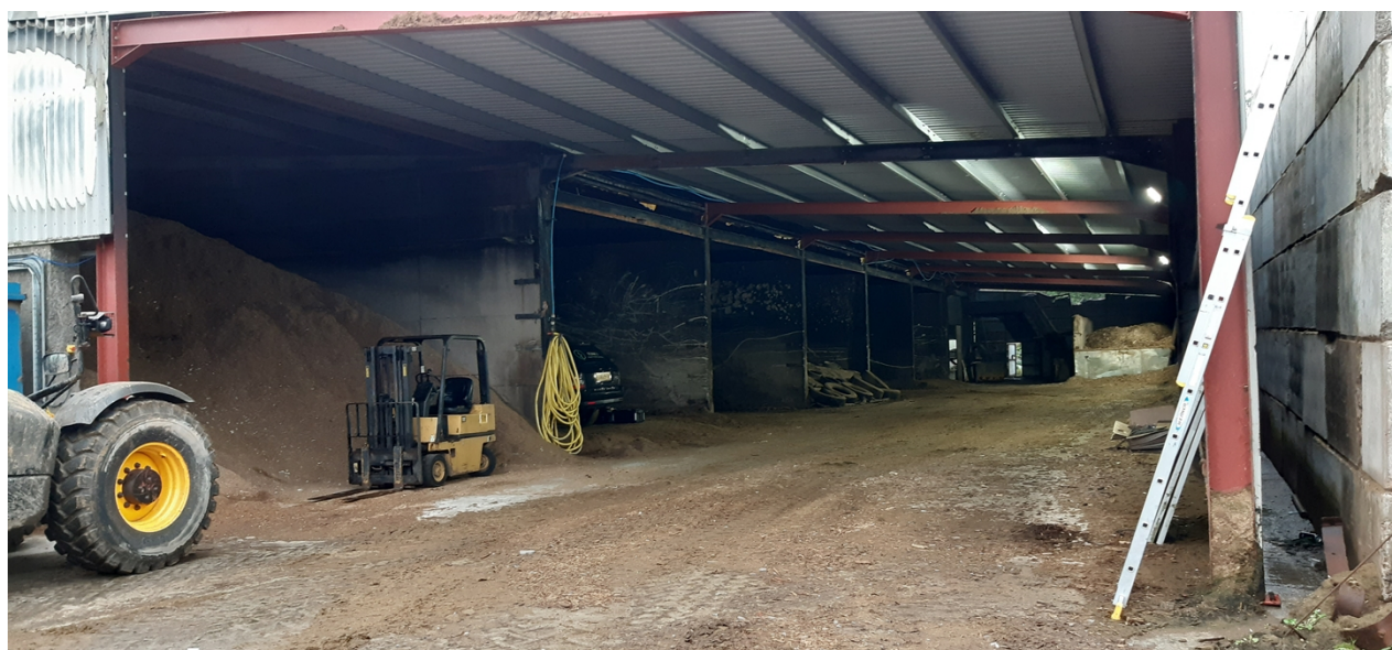
Photo 11 - Drying sheds area with infrastructure improvements taking place
