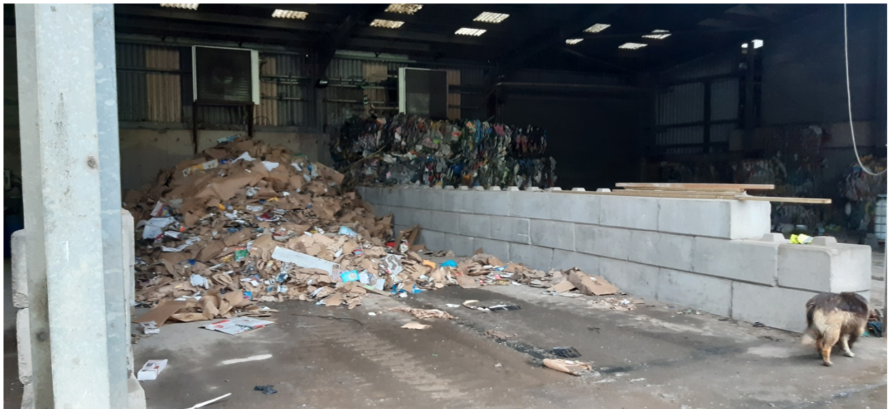
Photo 2 - View inside waste transfer station building
