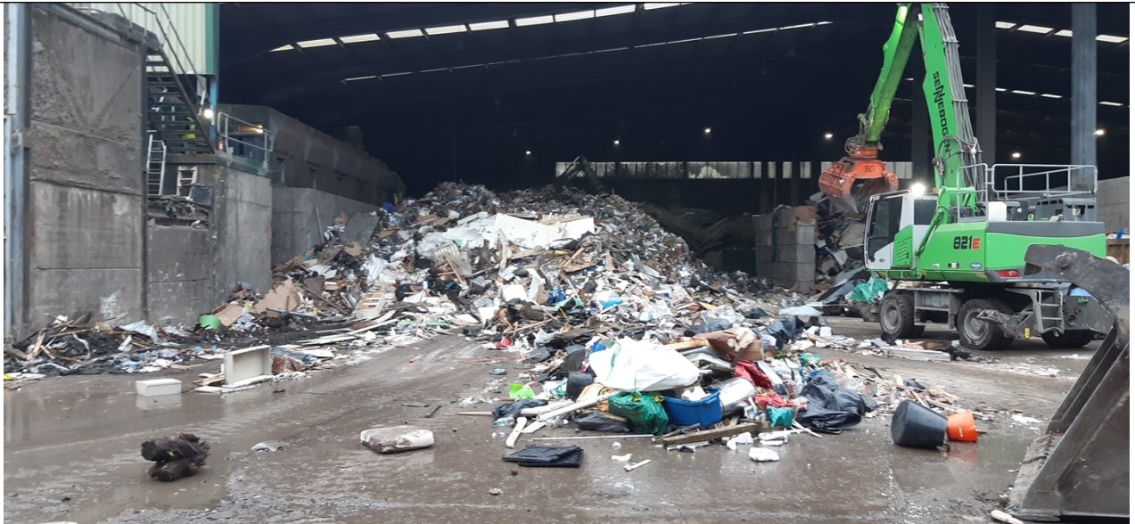
Photo 1 - View inside waste transfer station building
