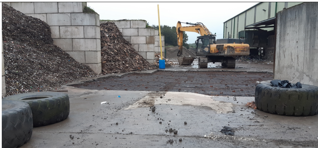
Photo 5 - Ongoing flooring infrastructure improvements at Bryn Recycling Ltd
