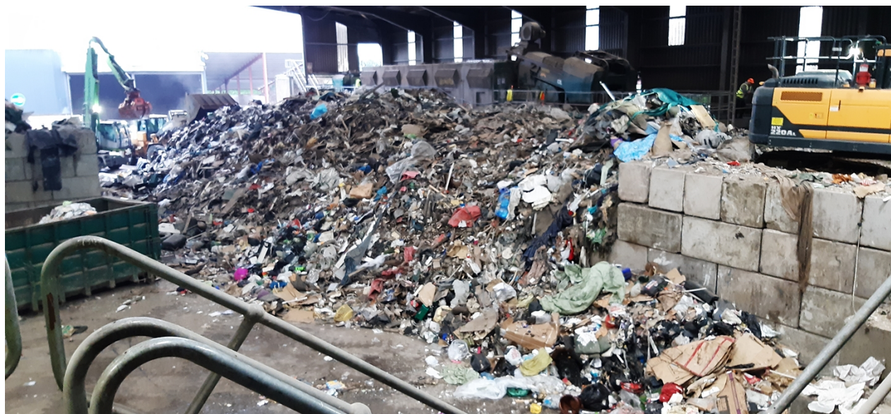
Photo 6 - Stockpile of waste(s) within waste transfer station
