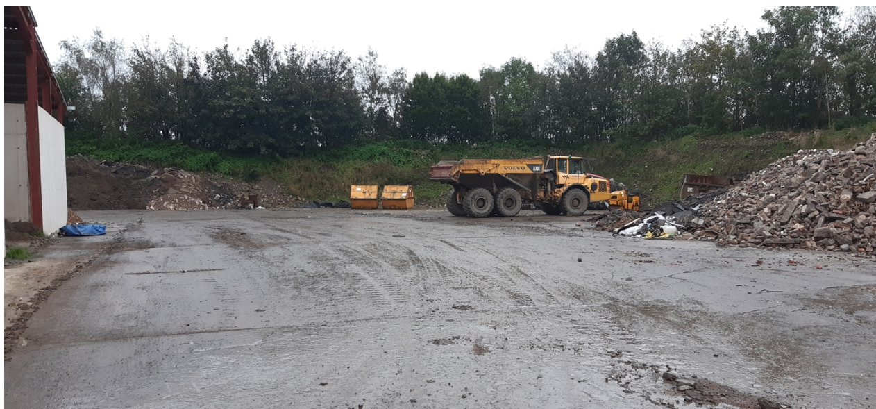
Photo 4 - Completed flooring infrastructure improvements at Bryn Recycling Ltd
