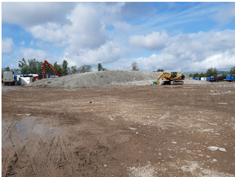
Picture 13 - Inert material with glass stockpile on Field 4
