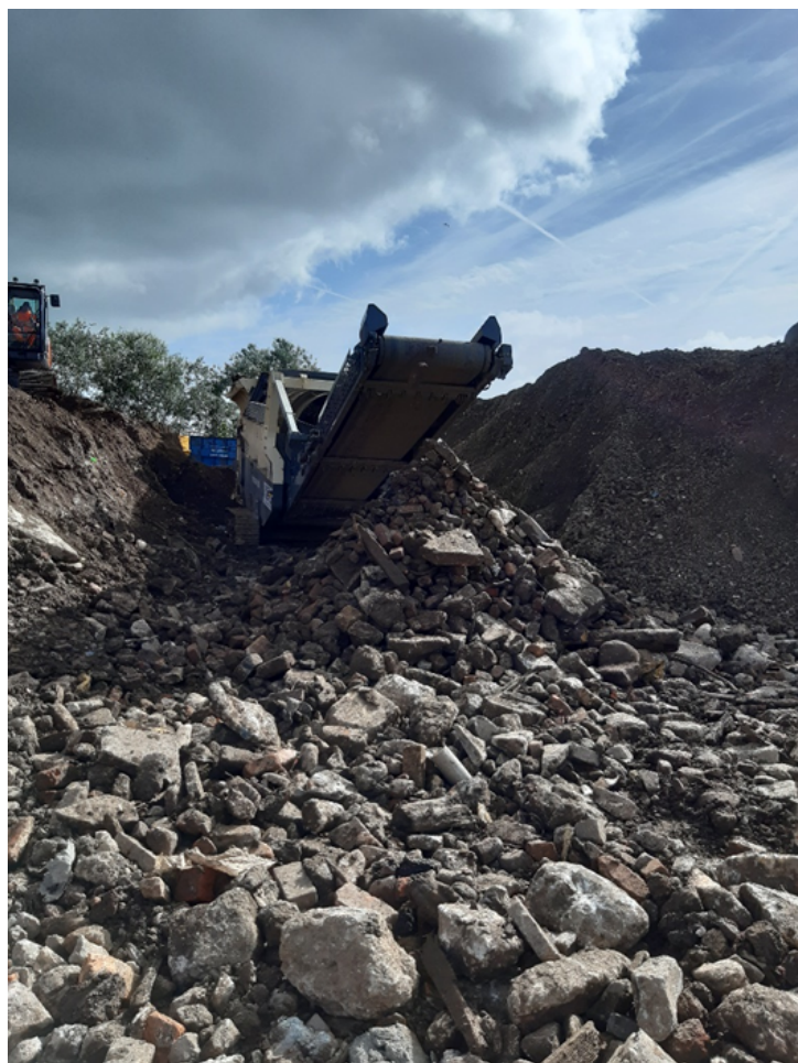
Picture 12 - Stone crusher in operation on Field 2
