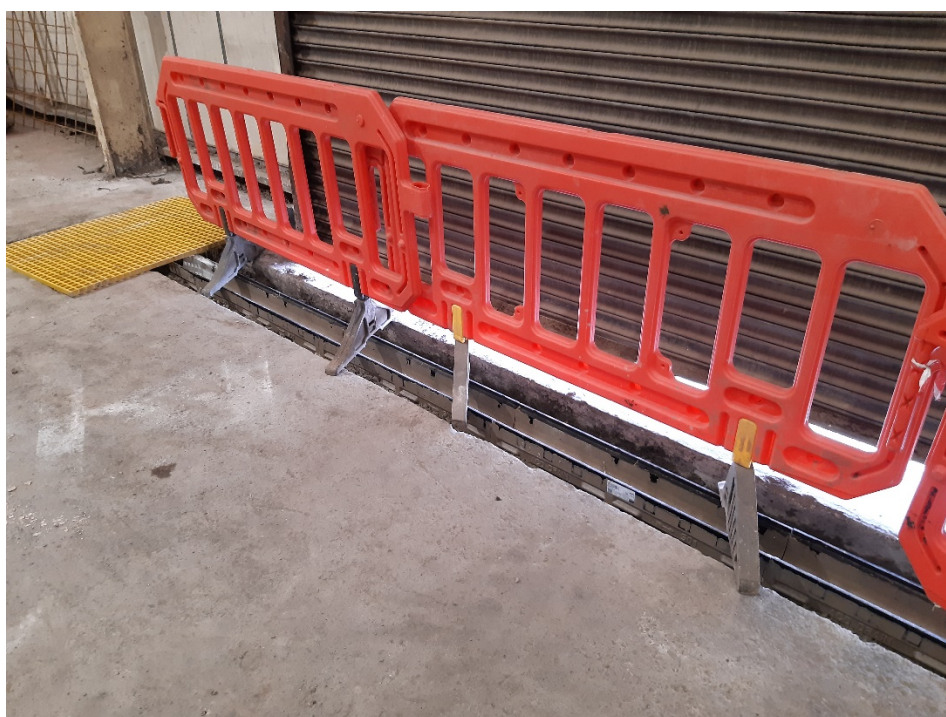
Photo 1 – newly installed channel strip drains along one of the entrances of Unit 5.
