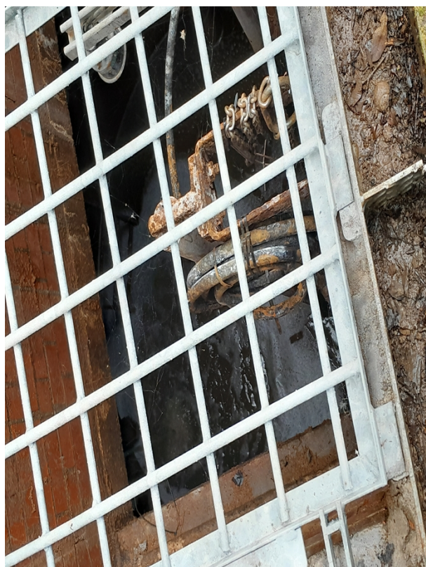
Gas Manifold - DSEAR Requirements need attention
