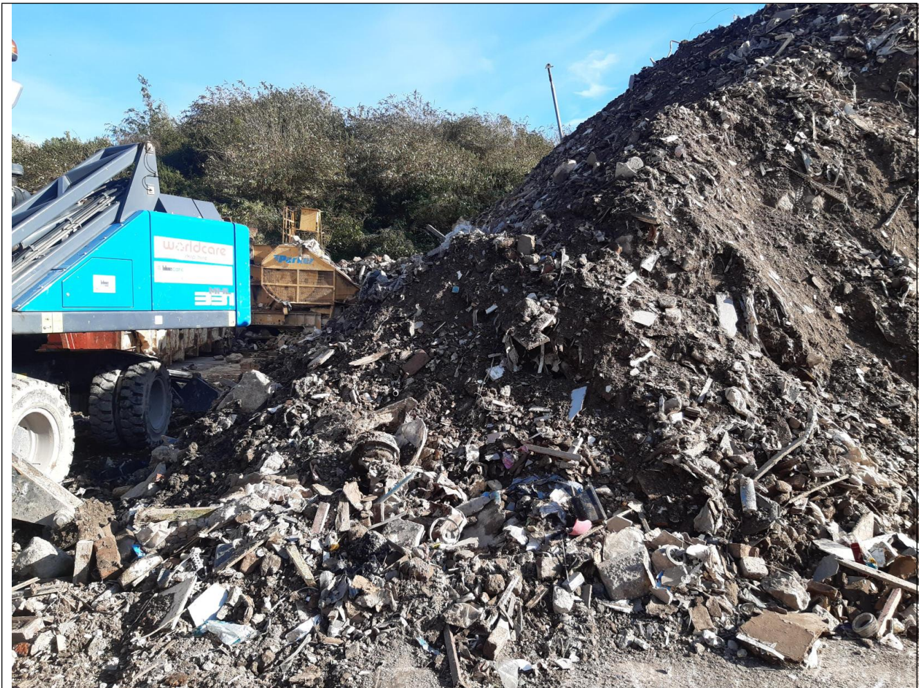
Photographs showing waste storage on site
